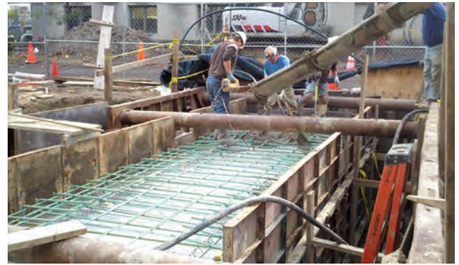
Fig. 4.1—Ready mixed concrete being placed. (Courtesy of Wiss, Janney, Elstner Associates, Inc.)
