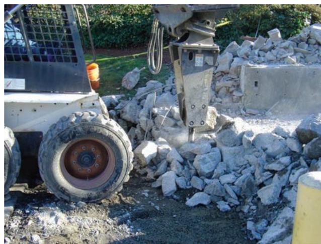
Fig. 3.2.4.2.2—Boom-mounted breaker.
