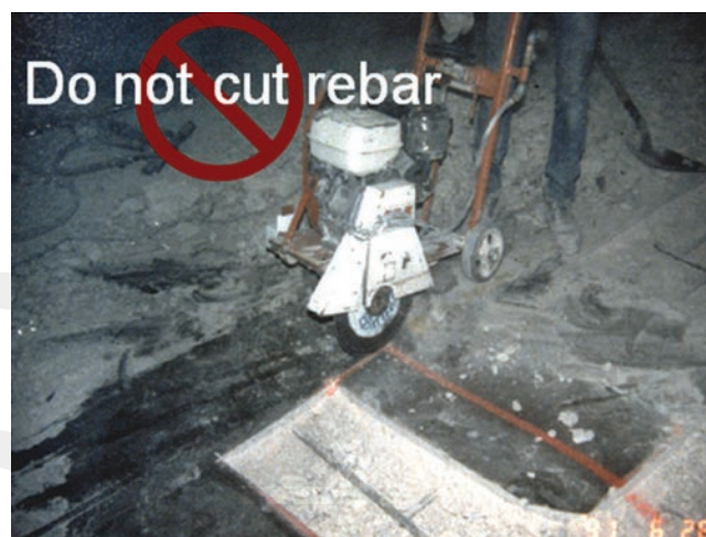
Fig. 3.2.2b—Saw cutting perimeter of repair area.
