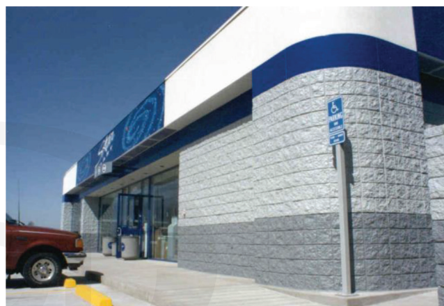
Fig. 3.1b—Standard flat and curved GFRP panels.
