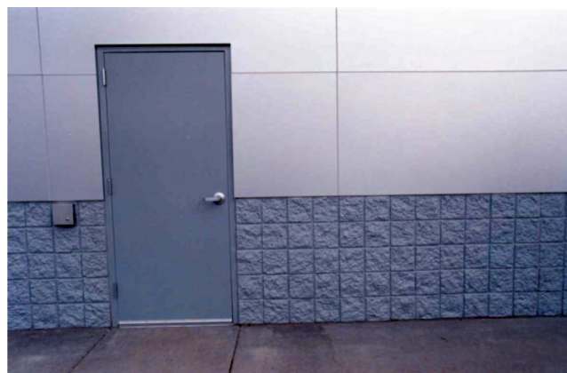
Fig. 3.1a—Standard GFRP panels with split-faced block finish.
