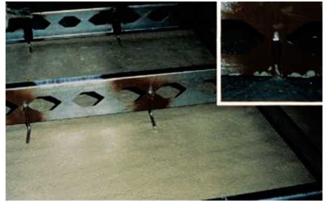
Fig. 3.1.1b—Flex-anchor connection with bond pad.
