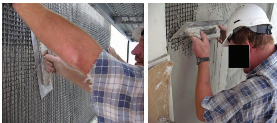
Fig. 4.2f—Strengthening of masonry walls by using a bidirectional carbon-fiber grid (0.6 x 0.6 in. [15 x 15 mm], having a mass per unit area of 4.03 lb/ft 2 [170 g/m 2 ] and an equivalent thickness of 0.0018 in. [0.047 mm]), applied with a fiber-reinforced pozzolan and cement mortar (courtesy of G&P Intech).
