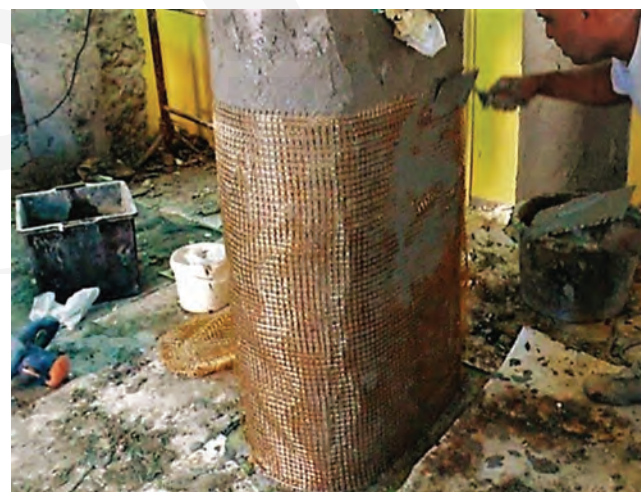
Fig. 4.4a—Seismic retrofit of a nursery in Zocca, Italy: confinement of columns (courtesy of Ruredil).
