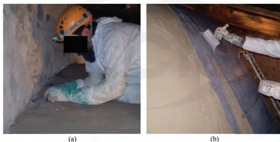
Fig. 4.3e—Strengthening intervention on the double curvature masonry bricks vault of S. Peter Apostle's Church in Giglio Island, Italy: (a) anchoring of the fabric; and (b) spreading of the primer (promoter of adhesion of the fabric to the matrix) (courtesy of Ardea).
