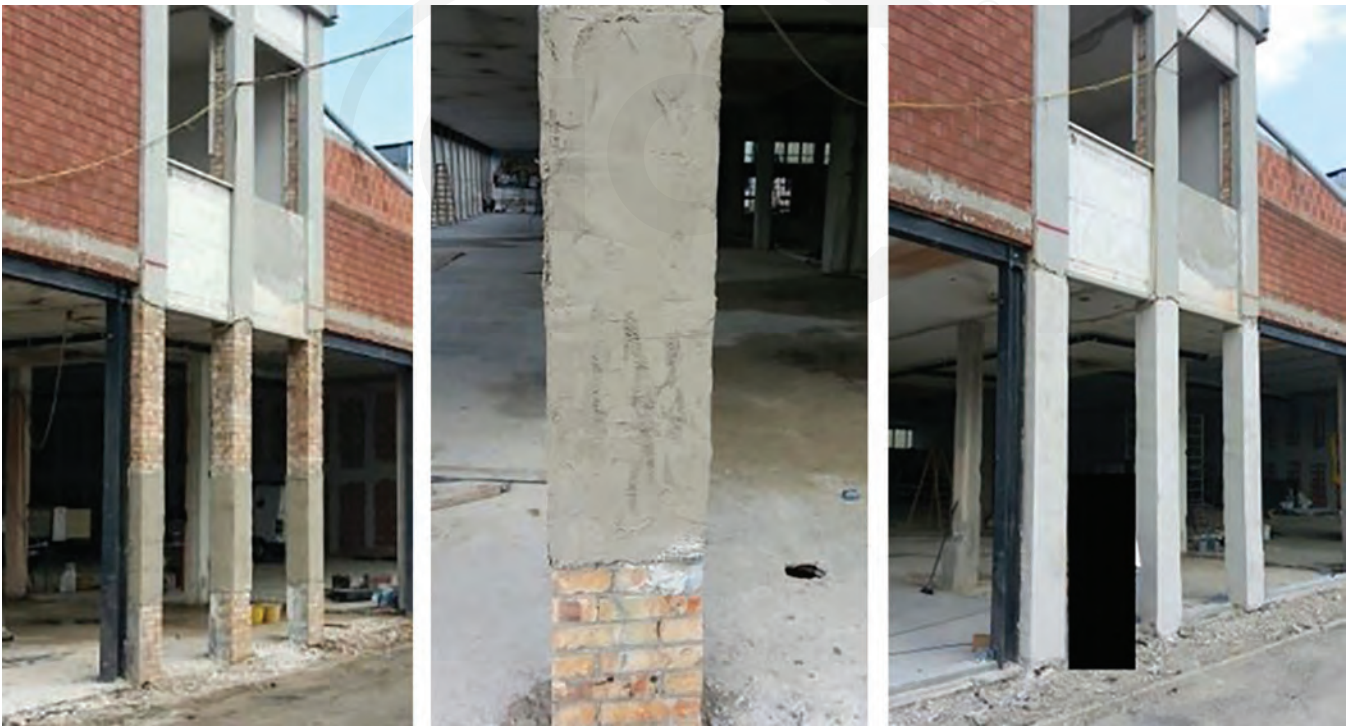
Fig. 4.4c—FRCM/SRG strengthening of masonry columns of the ex-bowling facility in Ravenna, Italy (courtesy of Kerakoll).
