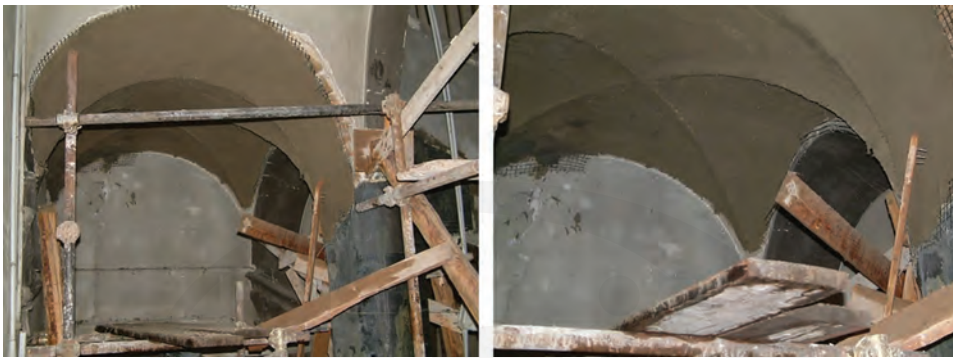
Fig. 4.3g—Strengthening of the intrados surface of a masonry vault, Italy. FRCM system is made up of a bidirectional fiber-glass fabric (1 x 1 in. [25 x 25 mm], 5.31 lb/ft 2 (225 g/m 2 ) mass per unit area) and cement-based mortar (courtesy of Mapei).
