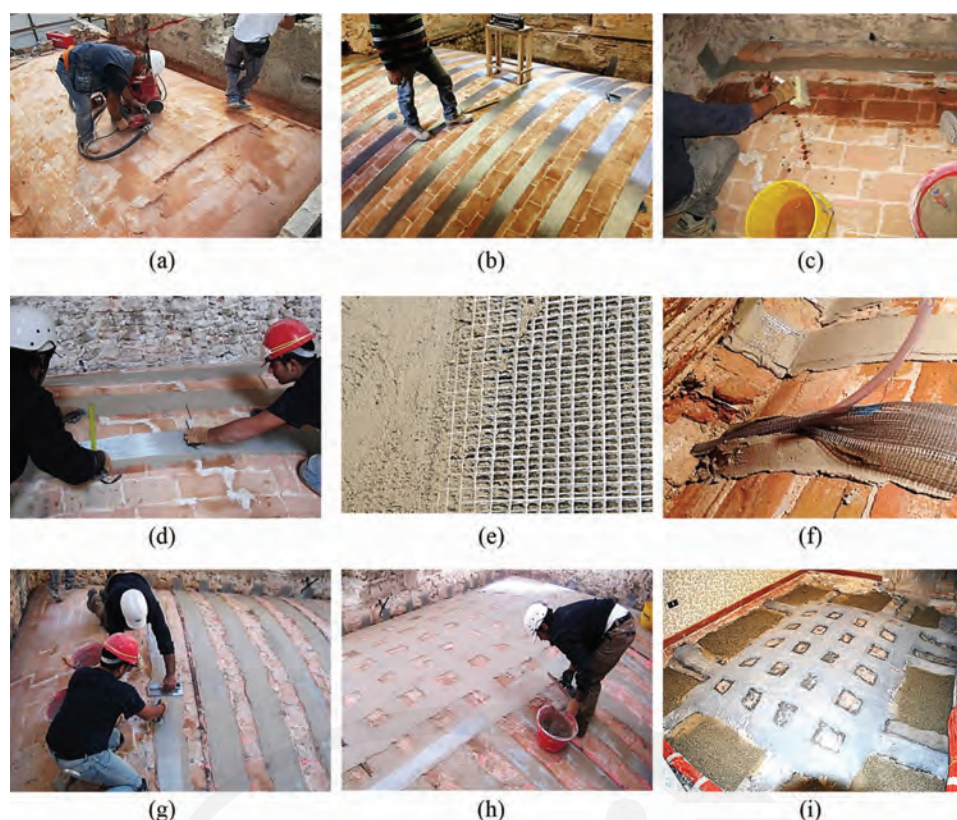
Fig. 4.3a—Application steps of a SRG system upon the extrados of a double curvature vault: (a) preparing of the vault surface; (b) cutting of the fabric strips; (c) wetting of the vault surface; (d) and (e) application of the fabric strips upon the first mortar layer; (f) preparation of the end connectors; (g) spreading of the top mortar layer; (h) installation of the transversal set of fabric strips; and (i) construction of buttresses and filling with granular material (courtesy of Cingoli).
