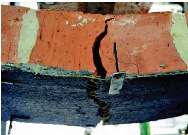
Fig. 3.4.1c—Failure by slippage of the PBO fabric within the matrix, followed by the tensile rupture of the fabrics (Carozzi et al. 2015).
