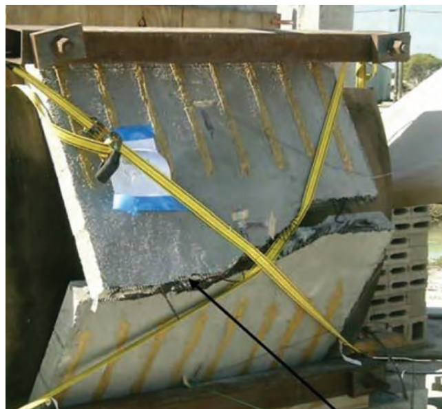
Fig. 3.4.1e—Failure by fabric slippage in the CMU wall panel (Babaeidarabad et al., 2014b).
