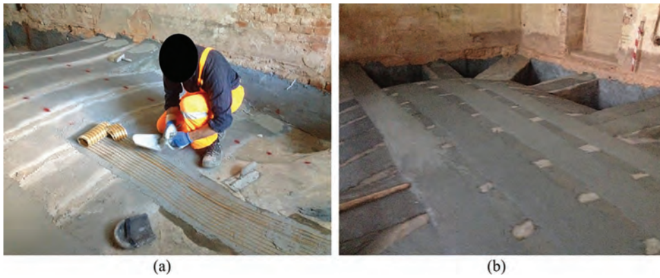
Fig. 4.3b—Strengthening intervention on a double curvature masonry vault of S. Andrea hospital in Vercelli, Italy, with PBO FRCM (courtesy of Cerutti).
