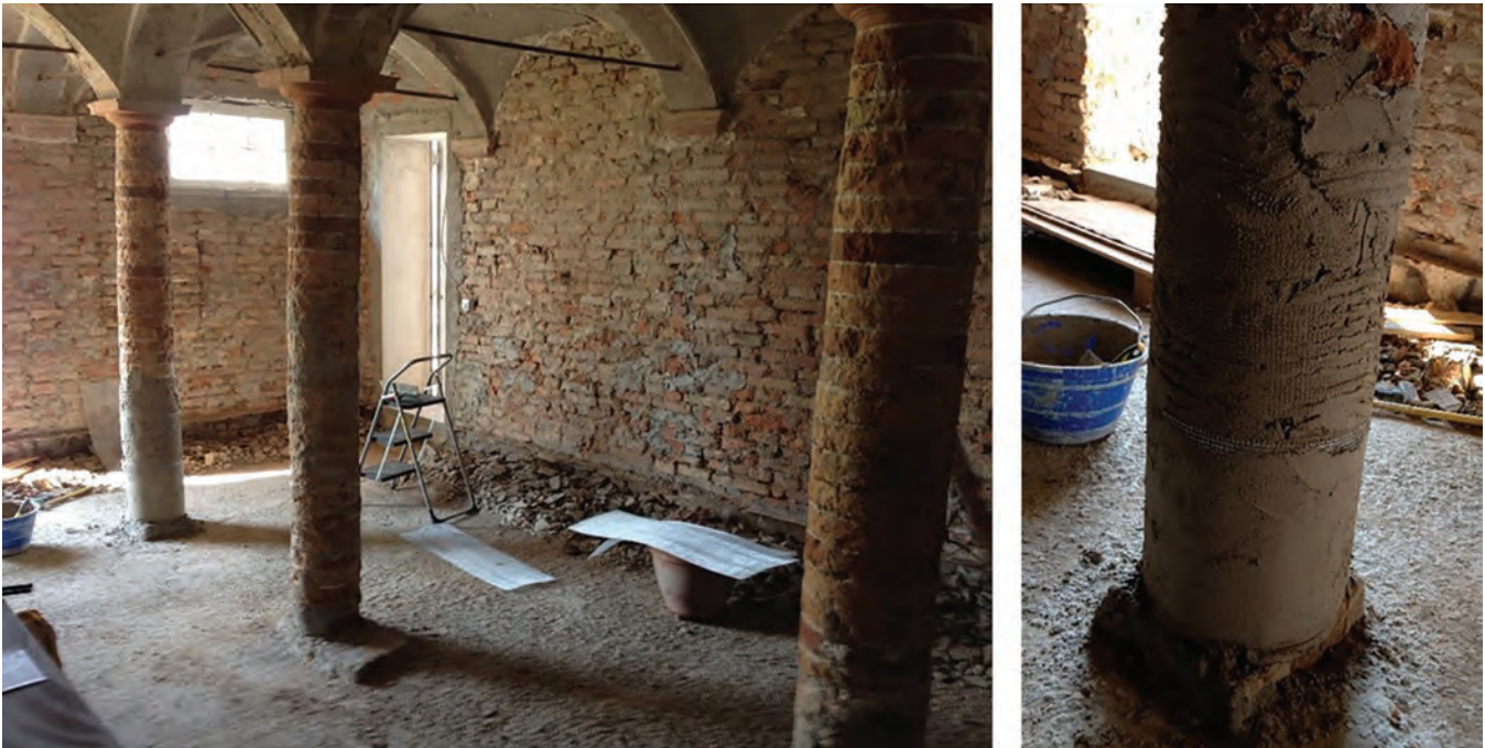
Fig. 4.4b—Columns confinement of a stable in Ravenna, Italy (courtesy of Kerakoll).
