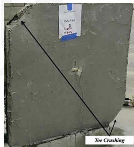
Fig. 3.4.2b—Crushing of the masonry panel reinforced with a carbon FRCM/SRG (Babaeidarabad et al. 2014a).
