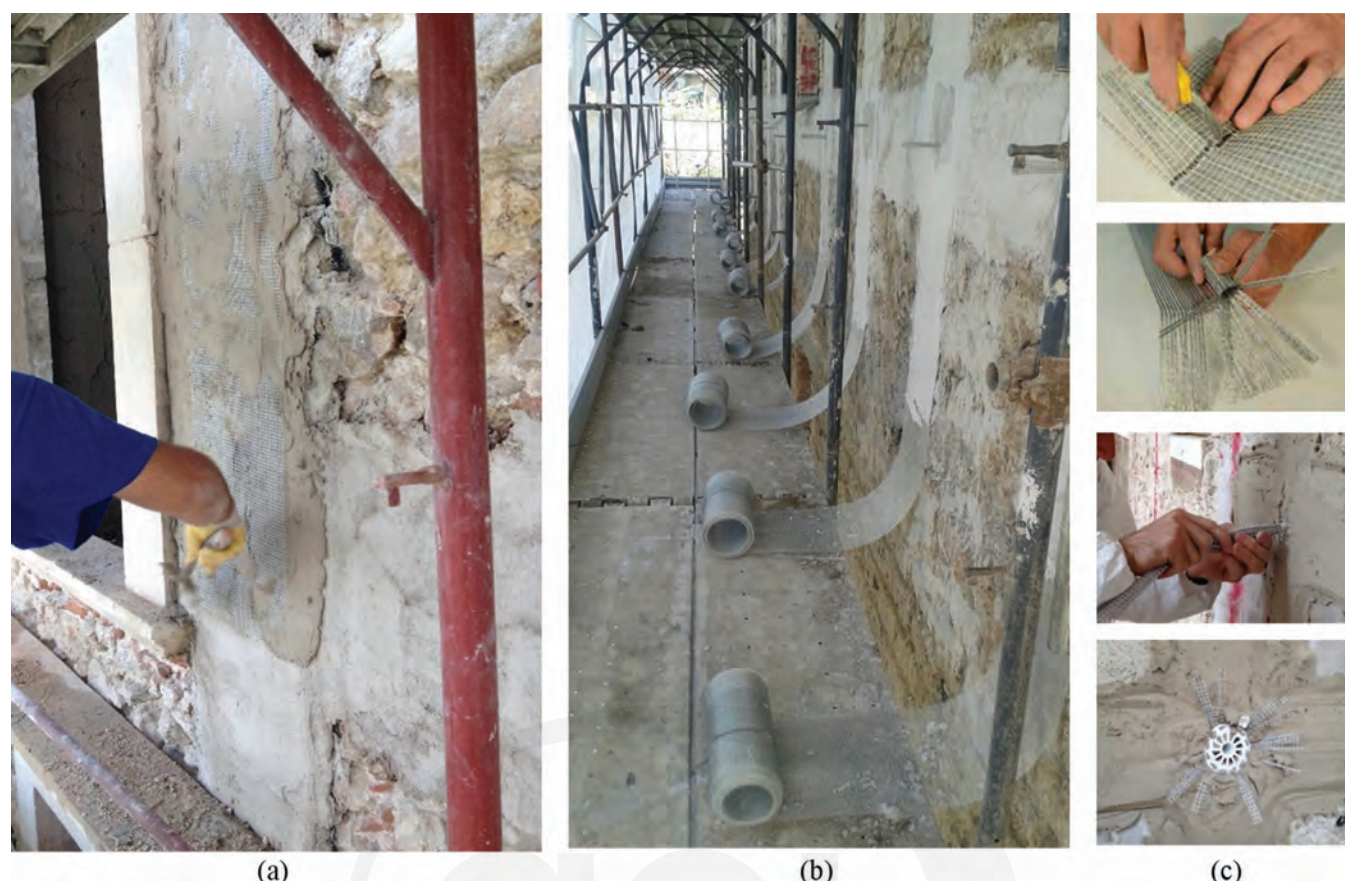
Fig. 4.2b—Retrofitting intervention with SRG on the application of unidirectional galvanized steel fabrics using lime based mortar and installation of mechanical connectors (courtesy of Kerakoll).
