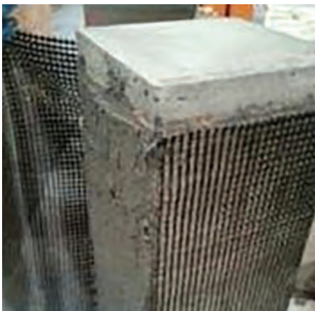
Fig. 3.4.3b—Installation of a carbon FRCM for confining a masonry column (Ombres et al. 2014).
