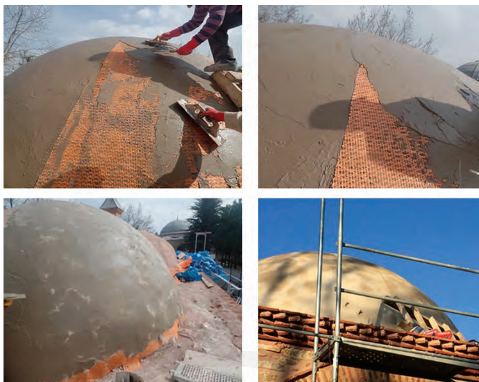
Fig. 4.3i—Strengthening intervention on a masonry dome of Sinanpasa Madrasa, Bursa, Turkey (courtesy of TICEM).
