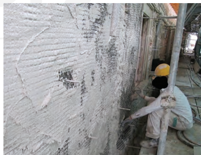
Fig. 4.2c—Strengthening of masonry walls with FRCM, Casino Ciolina, L'Aquila, Italy: application of a bidirectional glass fabric with lime-based mortar and spreading of the last layer of mortar (courtesy of Cingoli).
