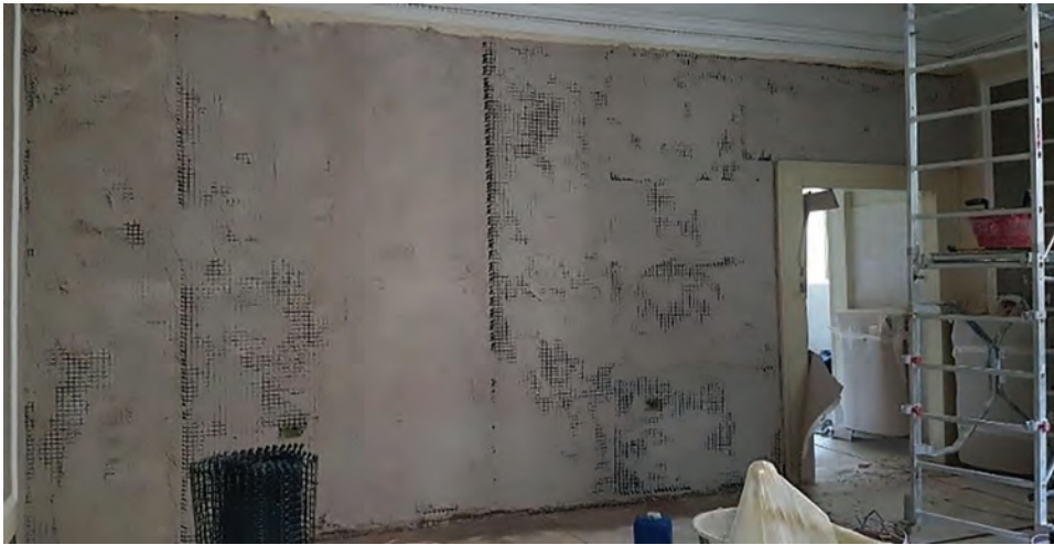
Fig. 4.2d—Common solution for the FRCM-strengthening of masonry walls against in-plane loads, Italy. System used: bidirectional fiberglass fabric (1 x 1 in. [25 x 25 mm], 5.34 lb/ft 2 [225 g/m 2 ] mass per unit area), embedded within an inorganic matrix (courtesy of Mapei).
