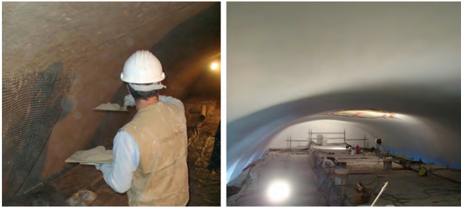
Fig. 4.3f—Strengthening of the masonry vaults of Santa Marta's Church (courtesy of S&P).
