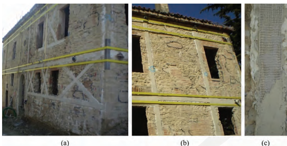
Fig. 4.2g—Seismic retrofitting of a damaged masonry building in San Marino: (a) in-plane and (b) out-of-plane strengthening of masonry walls; and (c) SRG details (courtesy of Kimia).
