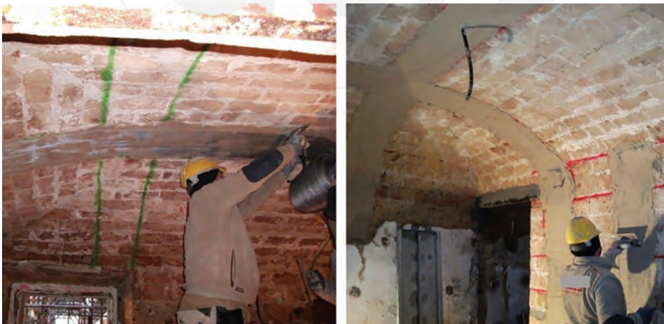
Fig. 4.3h—Strengthening of a masonry vault in L'Aquila, Italy. SRG system used: unidirectional galvanized steel fiber sheet (having a mass per unit area of 52.24 lb/ft 2 [2200 g/m 2 ] and an equivalent thickness of 0.0106 in. [0.27 mm]), applied with a lime-based mortar (courtesy of G&P Intech).
