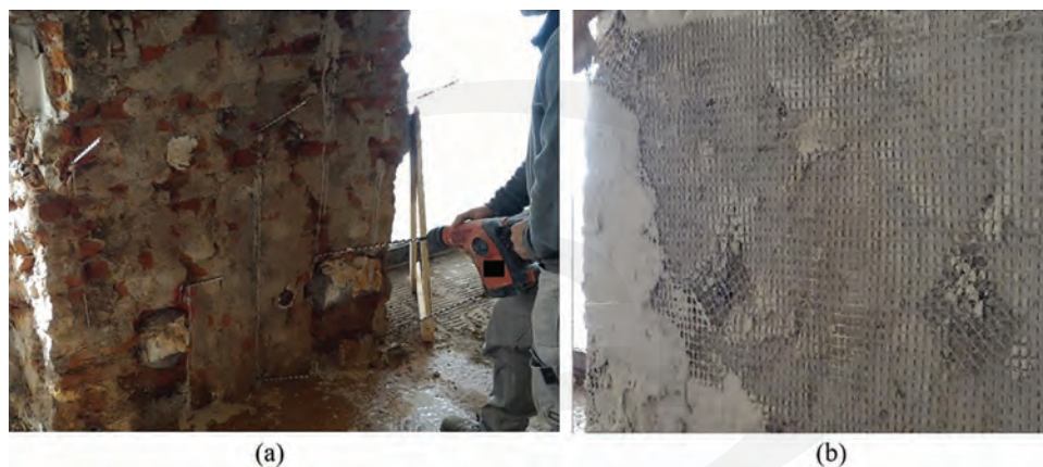
Fig. 4.2a—Strengthening of walls belonging to a damaged brick masonry building in Milan, Italy: (a) improving of the quality of masonry; and (b) application of the fabric (courtesy of TCS).
