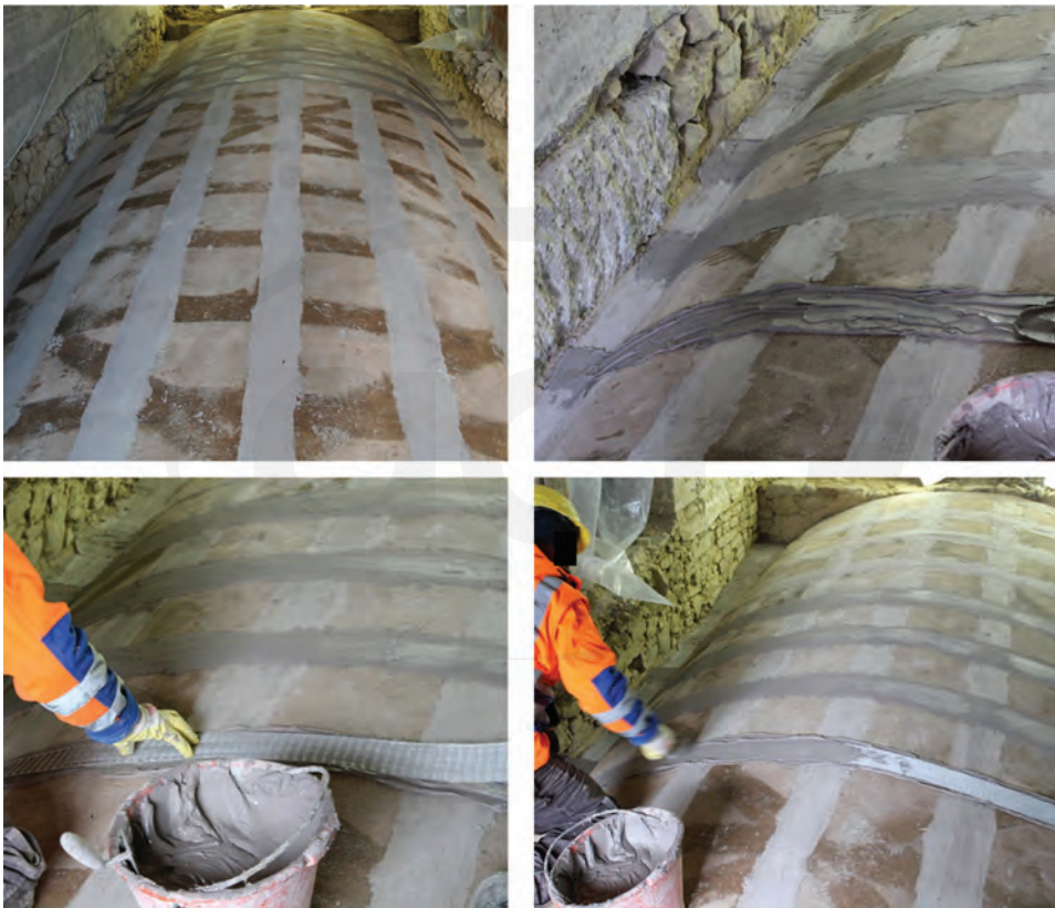
Fig. 4.3c—Seismic retrofitting of the stable of Santa Apollinare's fortress in Marsciano, Italy: strengthening of a masonry vault (courtesy of Kimia).
