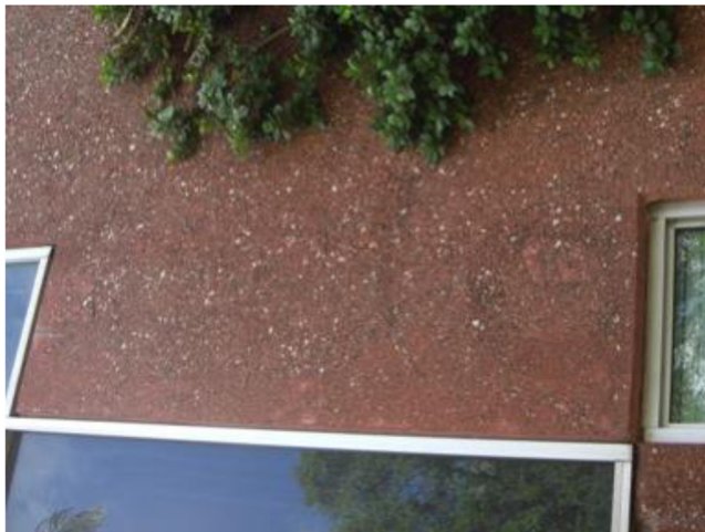
Fig. 3.2.3b—Detailed exposed aggregate finish.
