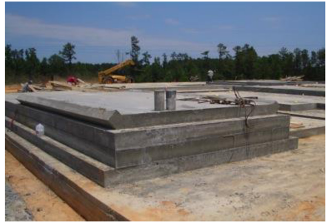
Fig. 4.9—Stack-cast panels.
