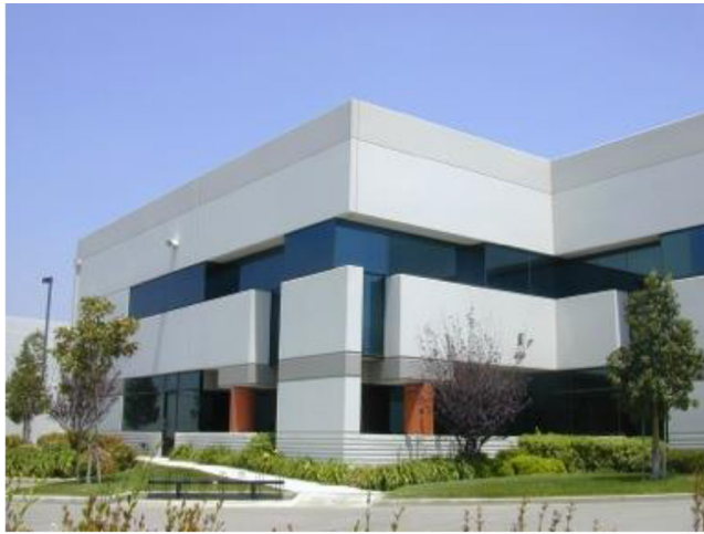
Fig. 3.2.3a—Tilt-up spandrel panels.
