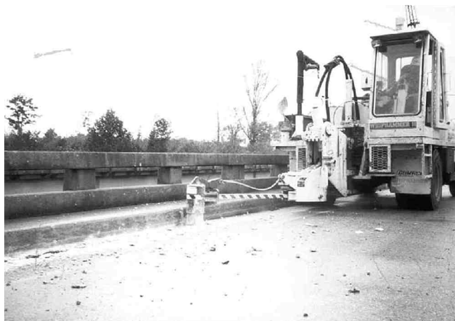
Fig. 3.3—Spring-action breaker (bridge deck demolition).
