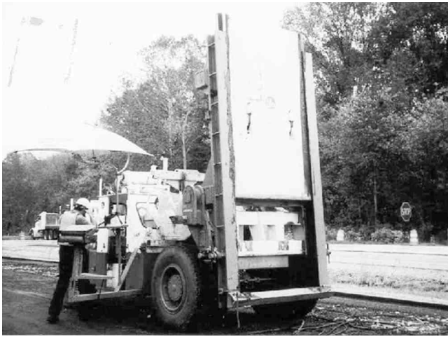
Fig. 3.1—Drop blade (highway pavement demolition).
