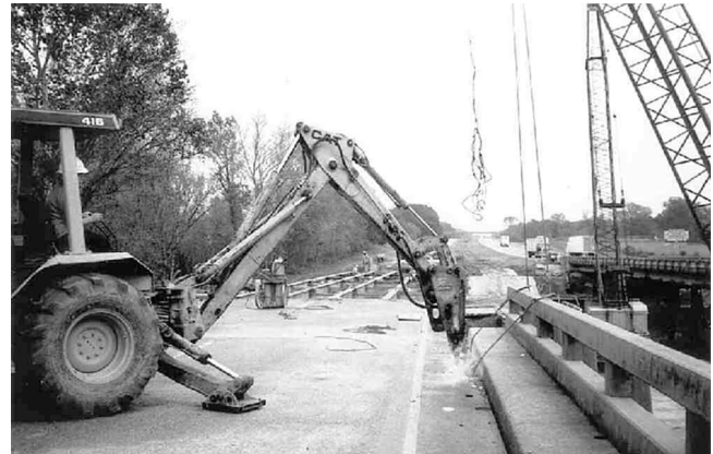
Fig. 3.2—Vehicle-mounted impact breaker (bridge deck demolition).
