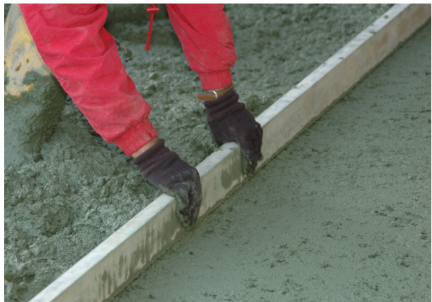
Fig. 1.1—Concrete is not delivered in its final form. The fresh concrete should be placed, consolidated, finished, and cured
