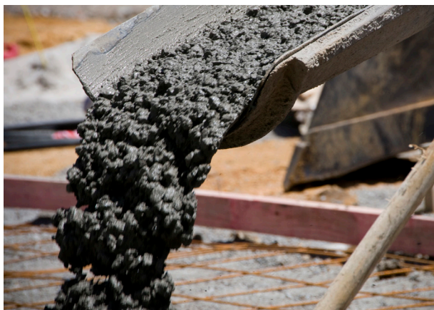
Fig. 1.8—Concrete discharging from a ready mixed concrete truck chute; each aggregate particle is coated with paste
