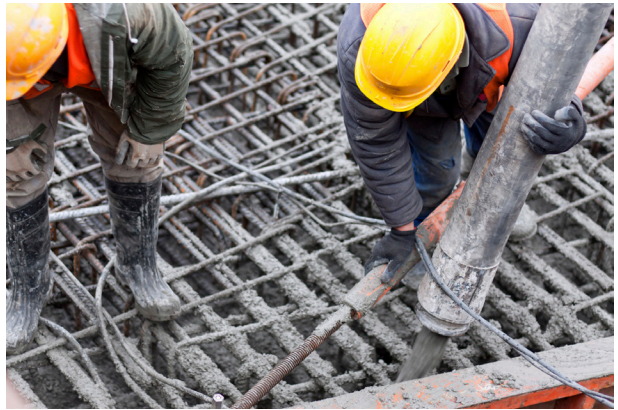
Fig. 2.1—Concrete workers placing concrete through reinforcement
