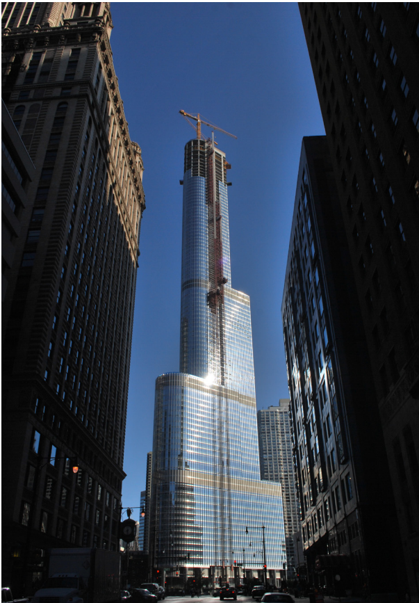
Fig. 1.6—Construction of the Trump International Hotel and Tower; Chicago, IL (photo courtesy of Lawrence Novak (PCA))
