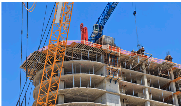
Fig. 1.7—Construction of a commercial skyscraper hotel in Dallas, TX
