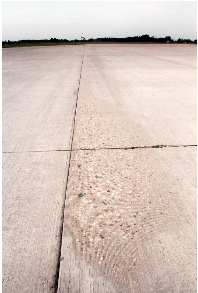
Fig. 0.5—Scaling removes the top layer of paste from the concrete (photo courtesy of PCA)
