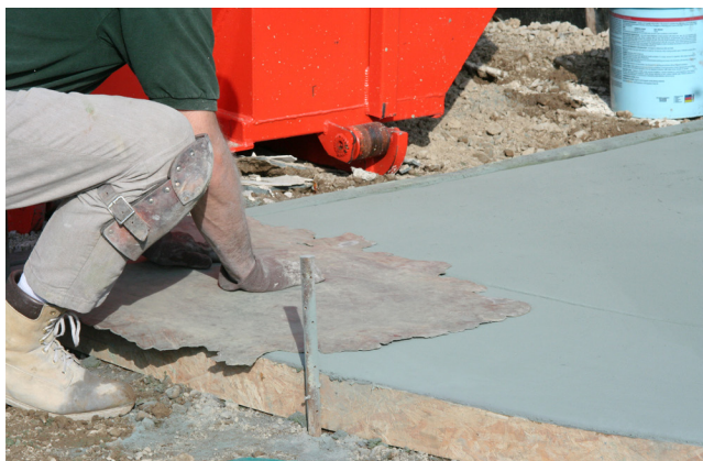
Fig. 1.12—Worker wearing knee pads to protect his skin from fresh concrete
