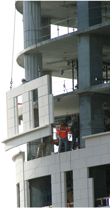
Fig. 1.2—Precast panel construction
