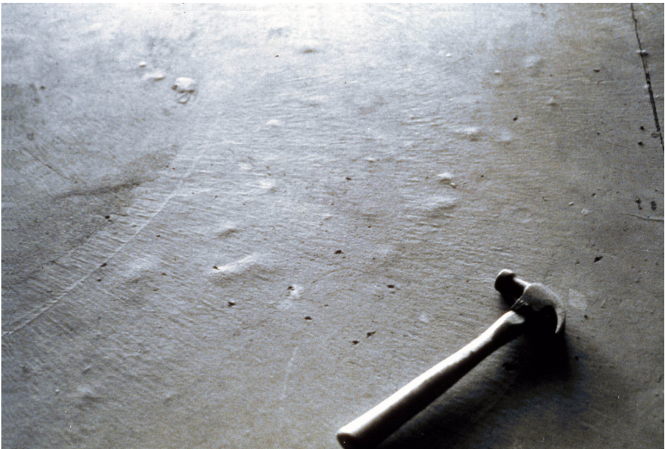
Fig. 0.2—Example of concrete surface blistering (photo courtesy of Portland Cement Association (PCA))
