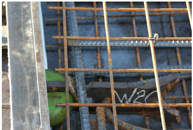
Fig. 2.2—Welded wire reinforcement
