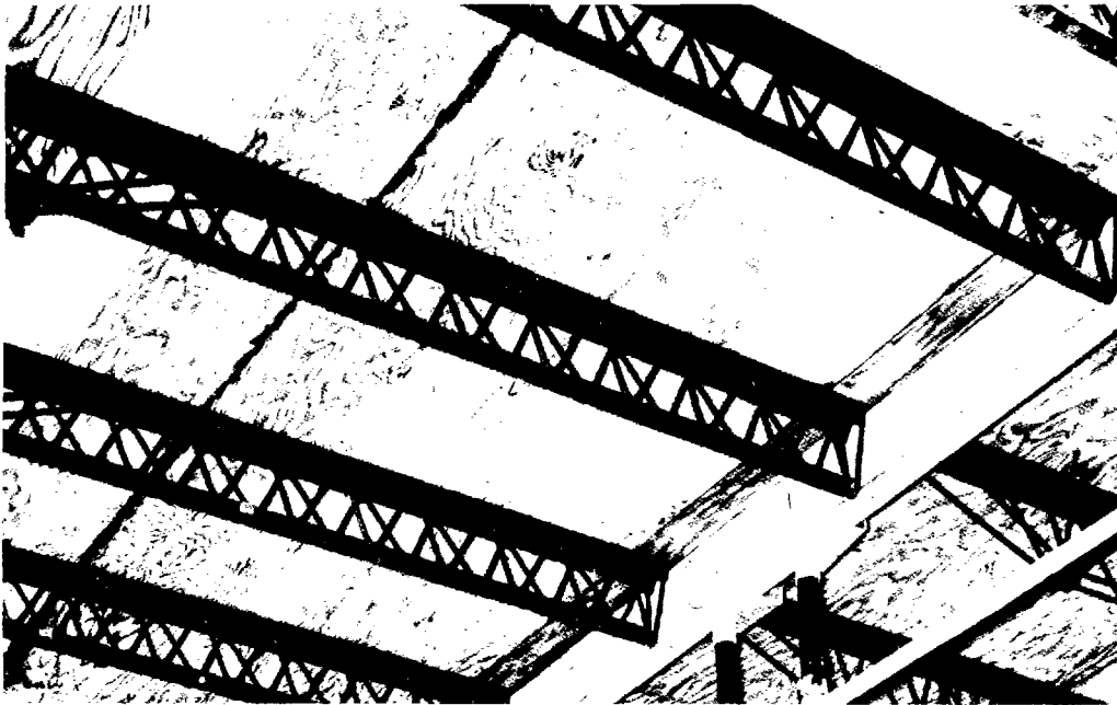
Fig. 3.7a—Plywood laid directly on typical telescoping lattice-type horizontal shoring to support concrete slab
