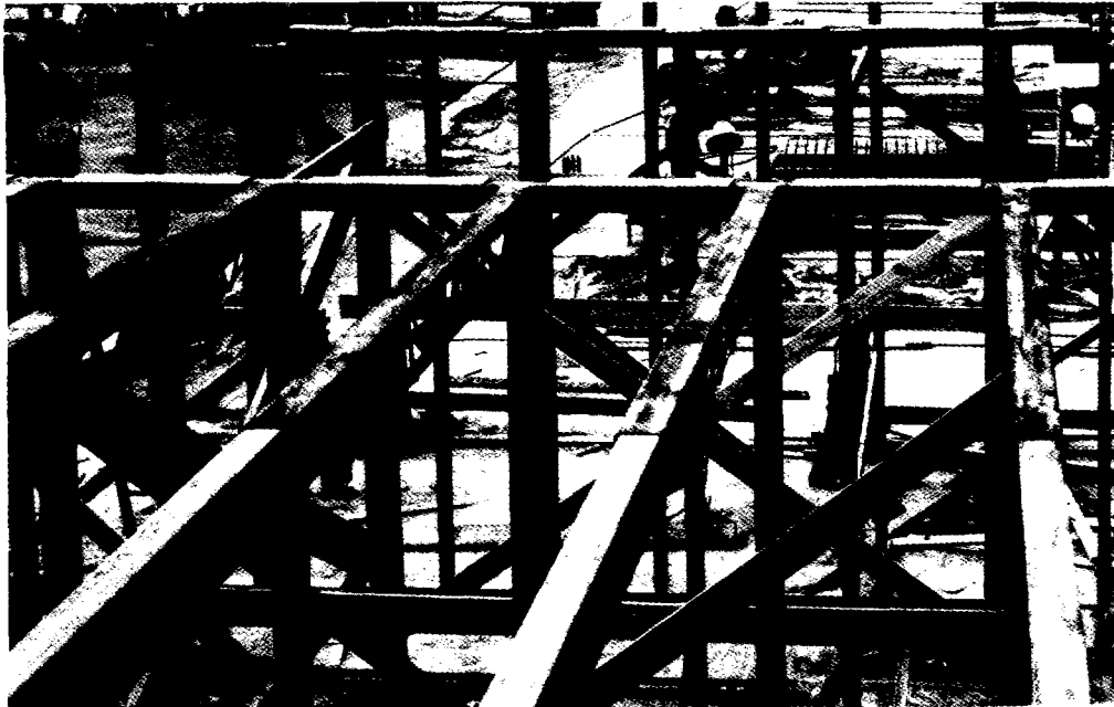
Fig. 3.7b—Horizontal shoring supported on braced wood bents. Filler pieces laid on top of bents allow stripping of decking and horizontal shores, while leaving wood bents in position as support for the partially cured slab.
