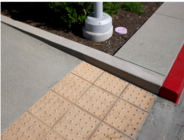
Fig. 2.10—Precast concrete truncated dome tiles at a handicapped access ramp
