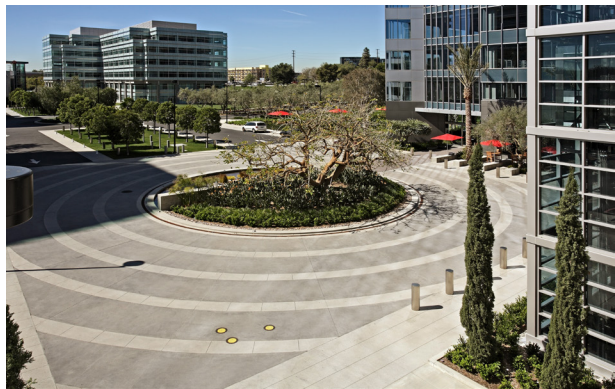
Fig. 4.2—Light gray concrete banding with dark gray concrete fields at a motor court
