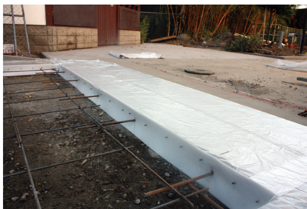
Fig. 4.5—Expansion joint material, steel dowels, and plastic sheeting for protection; ready for a concrete placement
