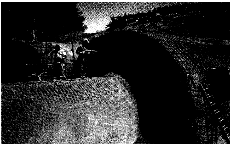
Shotcreting being performed from atop the portal structure.
