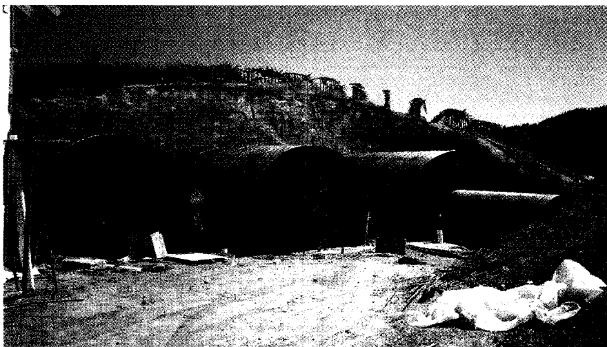
Completed plate shell structure.
