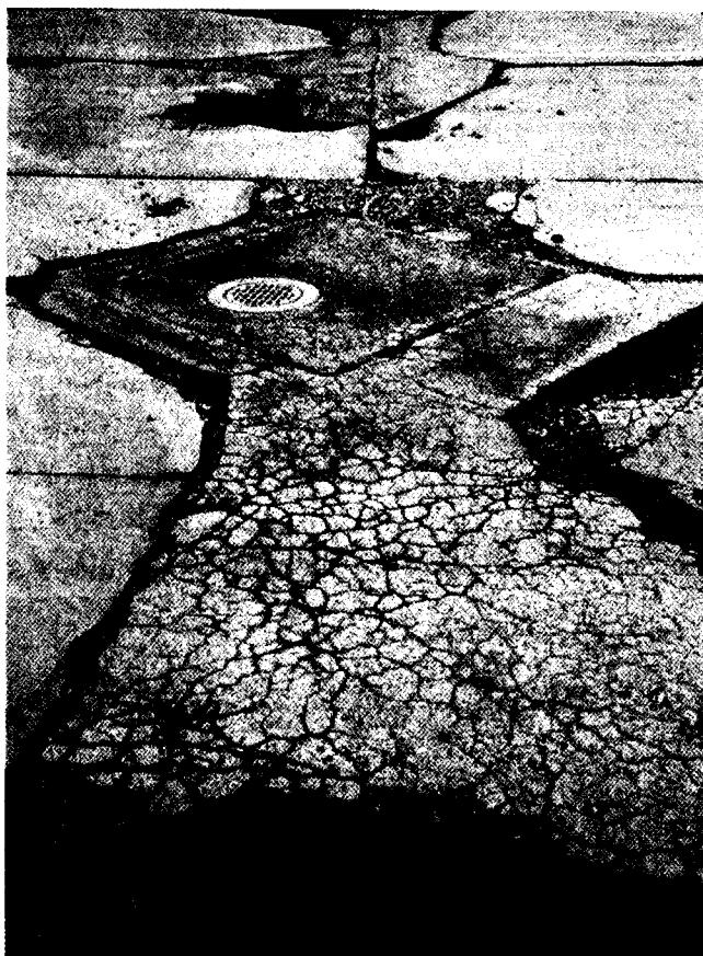
(left) Original condition of parking slab. (above) Suitability of the filter/separation layer in the drainage net system was evaluated in a trial installation.
