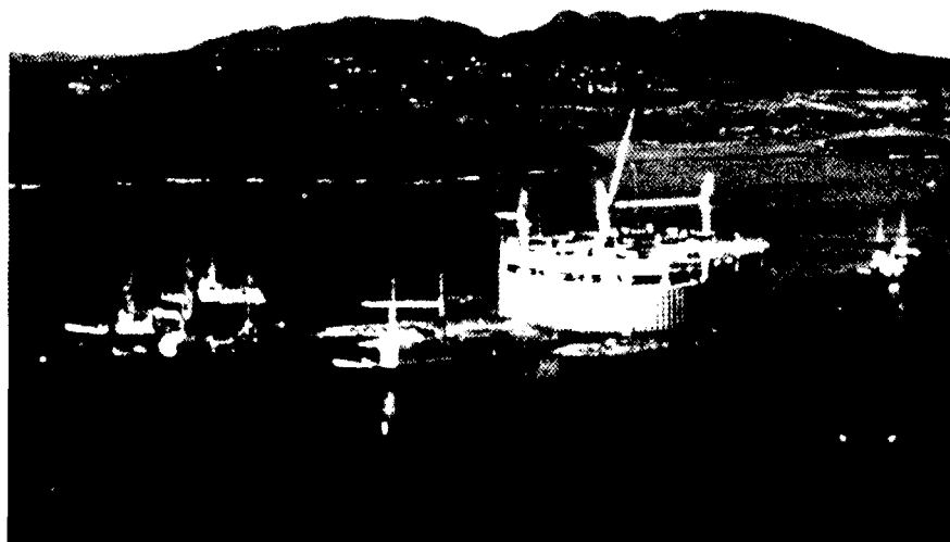
Fig. 1 — Oil tank under tow from Stavanger, Norway, to Ekofisk Field in the North Sea, Spring 1973.
