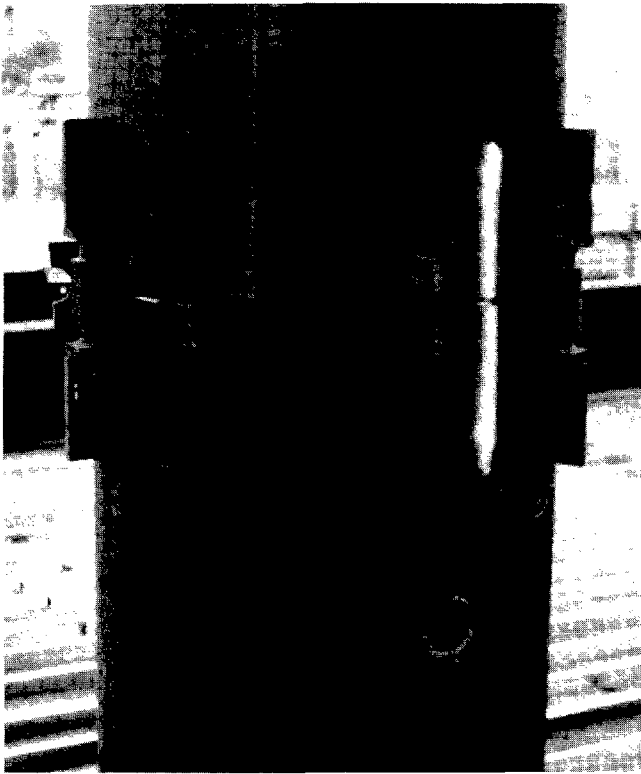
Fig. 5 — Splice between two tubular sections. Columns are supported temporarily on turnbuckles, which facilitate plumbing and alignment. The splice is completed by butt welding.
