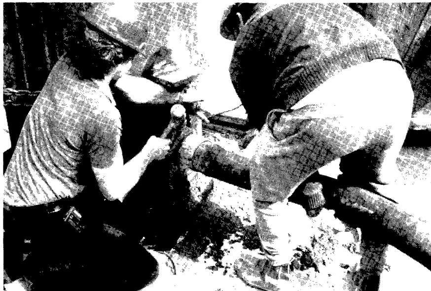
Fig. 4 — Concrete being placed into tubes at Casselden Place. A pump hose is connected to the base of the column and pumped up as far as six stories at a time. No vibration of the concrete or scabbling of the interface between placements is required.
