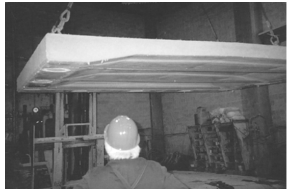
Fig. 3.5—Photograph showing straps embedded in an Arch-Panel.
