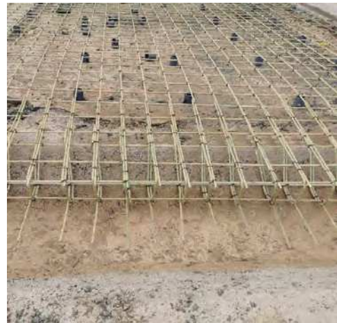
Fig. 1.2d—Currently the largest single project to use GFRP reinforcement, the Jizan Flood Mitigation Channel is a megaproject to protect the refining facilities of Saudi Aramco on the banks of the Red Sea in Saudi Arabia. The GFRP bar provides corrosion resistance in this coastal region and its light weight allowed for faster installation than traditional methods. There was a reported 21% cost savings in initial construction using GFRP bars versus epoxy-coated steel bars (Villen Salan et al. 2021).
