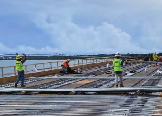
Fig. 1.2e—The Harker Island Bridge in Carteret County, NC, is a 3.2 mile (5 km) long vehicular bridge near the Outer Banks that includes 28 spans. The bridge deck is reinforced with GFRP bars, and the bridge girders are both prestressed with carbon FRP (CFRP) tendons and reinforced with GFRP bars. The entire bridge structure uses almost no steel reinforcement. FRP solutions were used on this bridge to combat the corrosive, brackish coastal environment of the Outer Banks.
