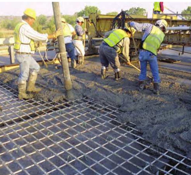
Fig. 1.1b—Bridge decks reinforced with GFRP bars as a way of mitigating corrosion issues when exposed to deicing salts. The photo on the left is of the Sierrita de la Cruz Creek Bridge in Amarillo, TX, which was constructed in 2000. The photo on the right is of the Red River Floodway bridge in Winnipeg, MB, Canada, which consumed over 310,000 lb (140,000 kg) of GFRP reinforcing bars and was constructed in 2006.
