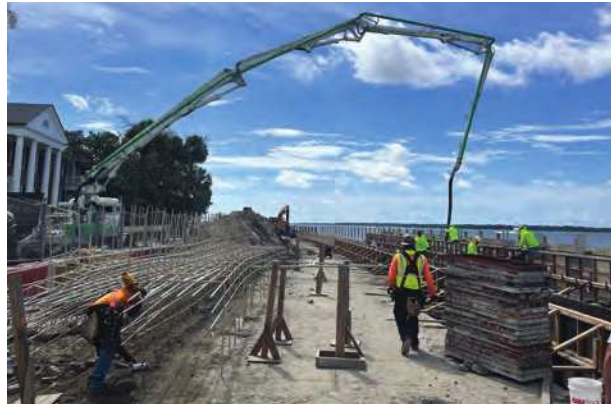
Fig. 1.2c—The Low Battery Seawall and seaside promenade is a historic landmark in Charleston, SC. The seawall was raised 1.8 ft (0.5 m) to match the High Battery Seawall. GFRP reinforcement was used due to its ability to resist corrosion in this severe coastal environment and for aesthetic concerns with steel corrosion products leaching onto the surface of the concrete (Steputat et al. 2022).
