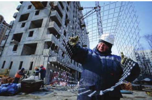
Fig. 2.2c—FRP grids used similarly to welded wire fabric for reinforcement of concrete slabs, walls, and other elements (photos courtesy Galen-Panamerica/Binevi)
