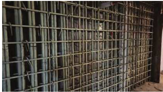
Fig. 1.2b—The foundations and shear walls of this eight-story building were reinforced with GFRP reinforcing bars. Sizes ranging from No. 3 to No. 11 bars were used and required complicated bend geometries for anchorages and ties. This illustrates the utility of GFRP bars in complex and demanding structural applications.
