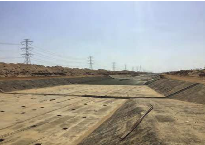
Fig. 1.2d—Currently the largest single project to use GFRP reinforcement, the Jizan Flood Mitigation Channel is a megaproject to protect the refining facilities of Saudi Aramco on the banks of the Red Sea in Saudi Arabia. The GFRP bar provides corrosion resistance in this coastal region and its light weight allowed for faster installation than traditional methods. There was a reported 21% cost savings in initial construction using GFRP bars versus epoxy-coated steel bars (Villen Salan et al. 2021).
