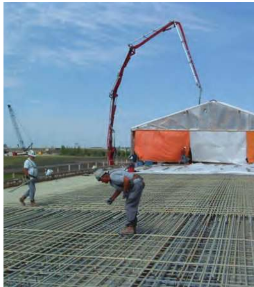
Fig. 1.1b—Bridge decks reinforced with GFRP bars as a way of mitigating corrosion issues when exposed to deicing salts. The photo on the left is of the Sierrita de la Cruz Creek Bridge in Amarillo, TX, which was constructed in 2000. The photo on the right is of the Red River Floodway bridge in Winnipeg, MB, Canada, which consumed over 310,000 lb (140,000 kg) of GFRP reinforcing bars and was constructed in 2006.
