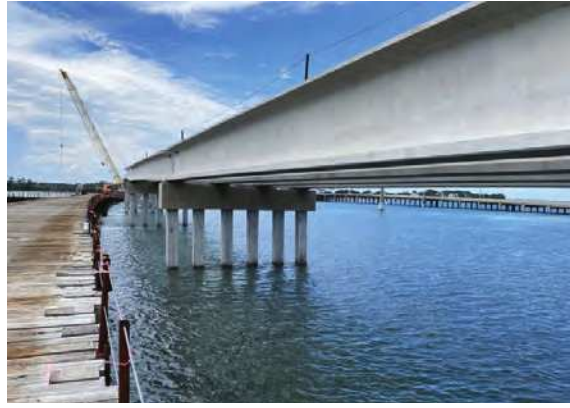
Fig. 1.2e—The Harker Island Bridge in Carteret County, NC, is a 3.2 mile (5 km) long vehicular bridge near the Outer Banks that includes 28 spans. The bridge deck is reinforced with GFRP bars, and the bridge girders are both prestressed with carbon FRP (CFRP) tendons and reinforced with GFRP bars. The entire bridge structure uses almost no steel reinforcement. FRP solutions were used on this bridge to combat the corrosive, brackish coastal environment of the Outer Banks.
