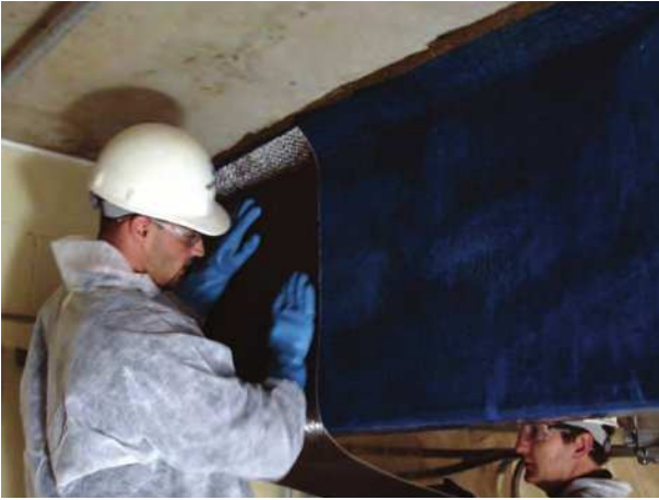
Fig. 2.2b—Externally bonded FRP reinforcement is often used to strengthen existing concrete elements. This photo shows a carbon fabric or wrap FRP system being applied with structural resins and adhesives to add external reinforcement to a concrete beam.
