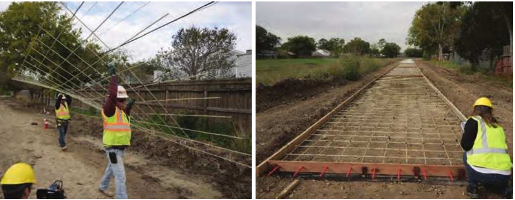
Fig. 1.2a—The use of GFRP reinforcing bars on Brays Bayou Hike & Bike Trail in Houston, TX, allowed the contractor to work efficiently using lighter equipment. This was in areas where heavier equipment was not always possible to use. The contractor was able to pre-tie grids of reinforcement that were easily moved into position.
