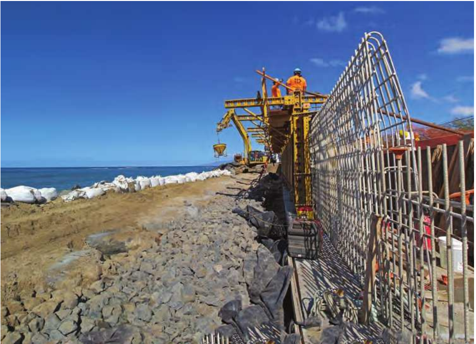
Fig 3.1.1b—GFRP reinforcement for a concrete seawall. Coastal structures such as this are highly susceptible to chloride-induced corrosion from seawater exposure. GFRP reinforcement provides a lasting solution for these applications (photo courtesy of Doug Green).
