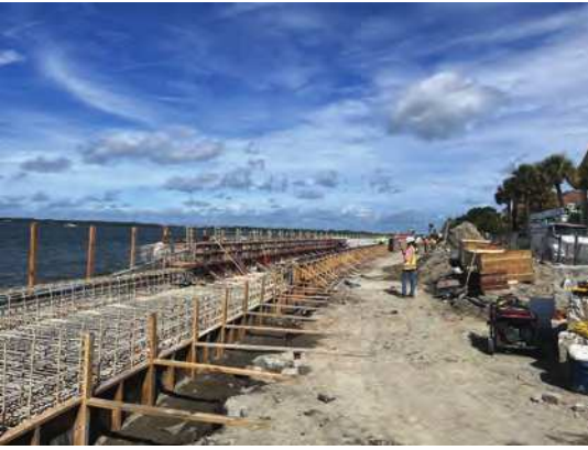
Fig. 1.2c—The Low Battery Seawall and seaside promenade is a historic landmark in Charleston, SC. The seawall was raised 1.8 ft (0.5 m) to match the High Battery Seawall. GFRP reinforcement was used due to its ability to resist corrosion in this severe coastal environment and for aesthetic concerns with steel corrosion products leaching onto the surface of the concrete (Steputat et al. 2022).
