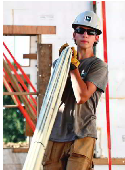
Fig. 3.3—A worker carrying a bundle of 12 No. 4 bars, 20 ft long. This bundle weighs less than 50 lb (photo courtesy MST Rebar, Inc.).
