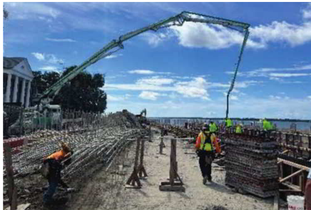
Fig. 5e—The Low Battery Seawall and seaside promenade is a historic landmark in Charleston, SC. The seawall was raised 1.8 ft (0.5 m) to match the High Battery Wall. GFRP reinforcement was used due to its ability to resist corrosion in this severe coastal environment and for aesthetic concerns with steel corrosion product leaching onto the surface of the concrete (Steputat et al. 2022).
