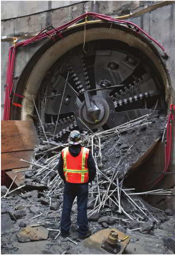
Fig 3.4b—A tunnel boring machine (TBM) exiting a “soft eye” reinforced with GFRP bars (photo courtesy of Owens Corning Infrastructure Solutions).
