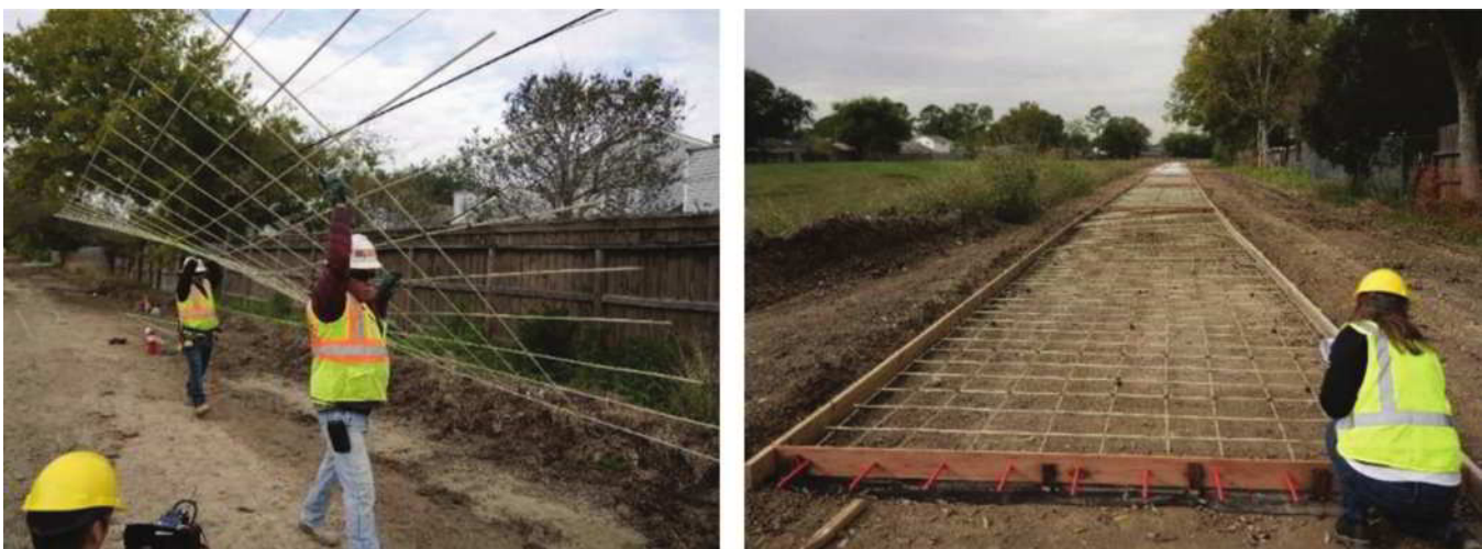
Fig. 5c—The use of GFRP reinforcing bars on Bray’s Bayou Hike & Bike Trail in Houston, TX, allowed the contractor to work efficiently using lighter equipment. This was in areas where heavier equipment was not always possible to use. The contractor was able to pre-tie grids of reinforcement that were easily moved into position.
