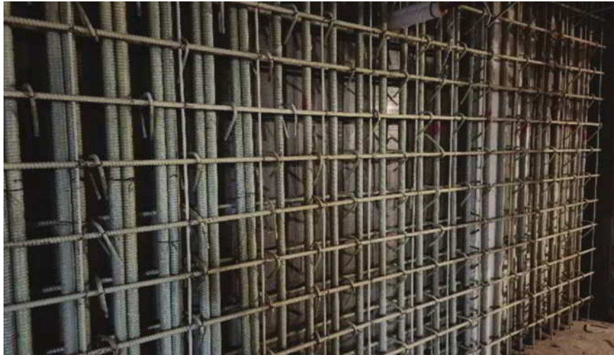
Fig. 5d—The foundations and shear walls of this eight-story building were reinforced with GFRP reinforcing bars. Sizes ranging from No. 3 to No. 11 bars were used and required complicated bend geometries for anchorages and ties. This illustrates the utility of GFRP bars in complex and demanding structural applications.
