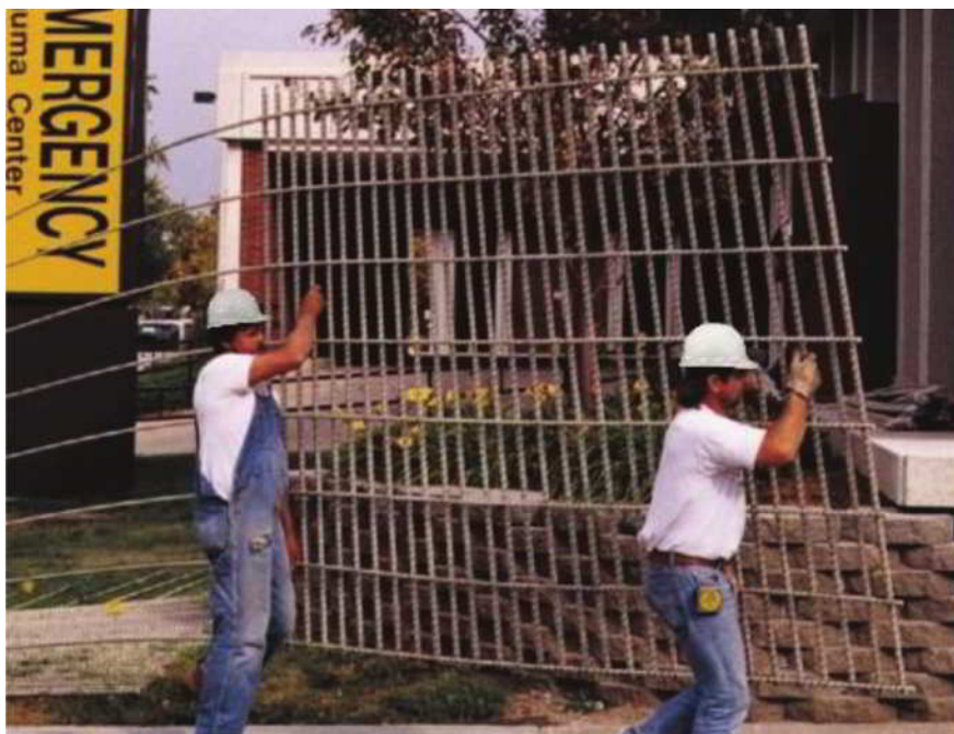
Fig. 5a—A GFRP reinforcement cage being transported to a concrete placement in a room that will eventually house an MRI unit (photo courtesy of Doug Gremel).
