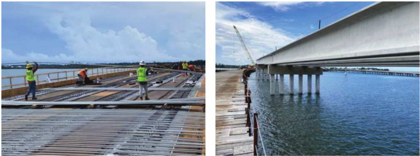
Fig. 5g—The Harker Island Bridge in Carteret County, NC, is a 3.2 mile-long vehicular bridge near the Outer Banks that includes 28 spans. The bridge deck is reinforced with GFRP bars, and the bridge girders are both prestressed with carbon FRP (CFRP) tendons and reinforced with GFRP bars. The entire bridge structure uses almost no steel reinforcement. FRP solutions were used on this bridge to combat the corrosive, brackish coastal environment of the Outer Banks.
