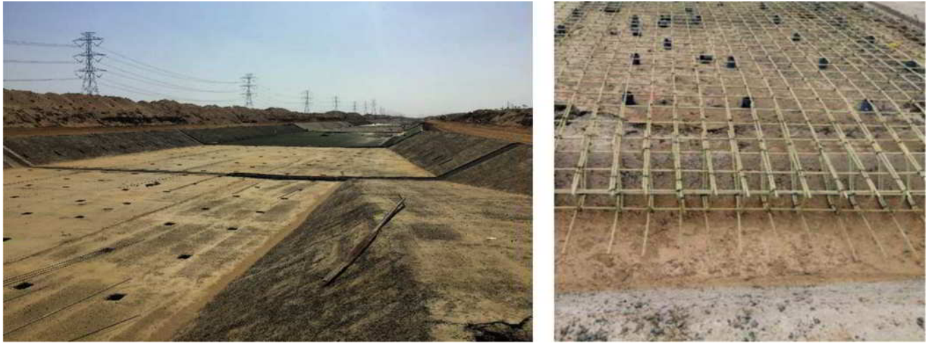
Fig. 5f—Currently the largest single project to use GFRP reinforcement, the Jizan Flood Mitigation Channel is a megaproject to protect the refining facilities of Saudi Aramco on the banks of the Red Sea in Saudi Arabia. The GFRP bar provides corrosion resistance in this coastal region and its light weight allowed for faster installation than traditional methods. There was a reported 21% cost savings in initial construction using GFRP bars versus epoxy-coated steel bars (Villen Salan et al. 2021).
