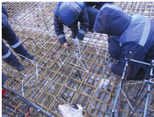
Fig. 3.7—Working with GFRP bars in cold conditions (photo courtesy of Galen-Panamerica/Binevir).
