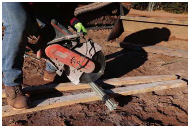
Fig. 3.4a—A bundle of GFRP bars being cut through on a job site (photo courtesy GatorBar).
