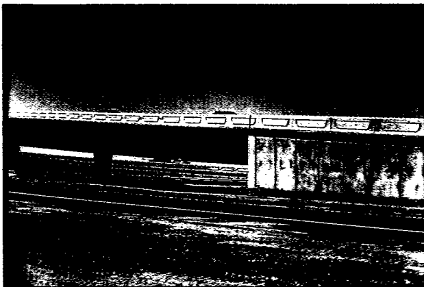
Fig. 8--San Francisco Airport viaduct abutment exposed aggregate
