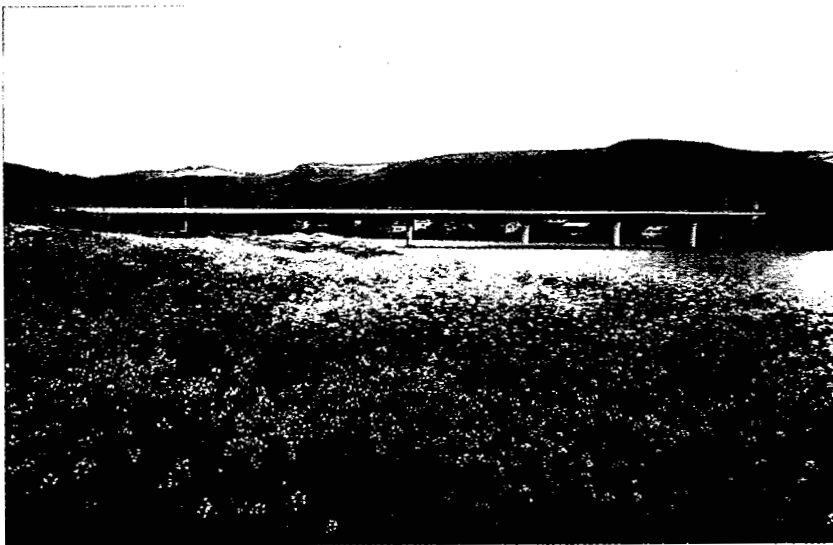
Fig. 10--New Russian River Bridge at Jenner
