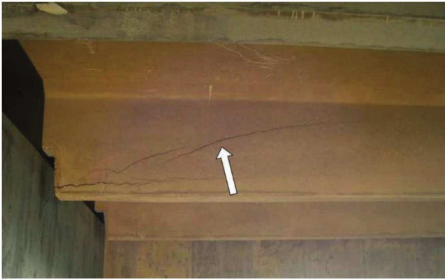
Fig. 4.1.2.3—Diagonal crack.
