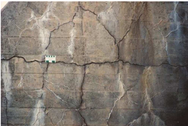
Fig. 4.1.2.5—Map cracking.
