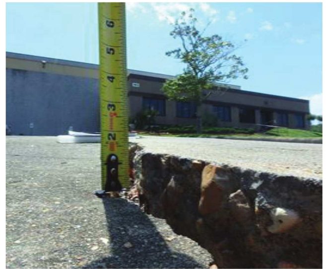
Fig. 4.2.5—Faulting.
