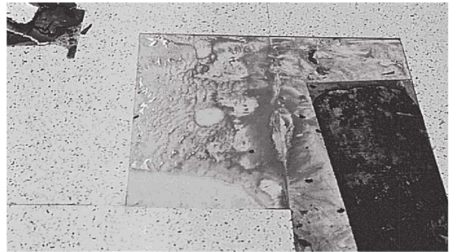
Fig. 1.3e—Adhesive degradation leading to debonded solid vinyl tile installed over asbestos tile (photo courtesy of P. Craig).
