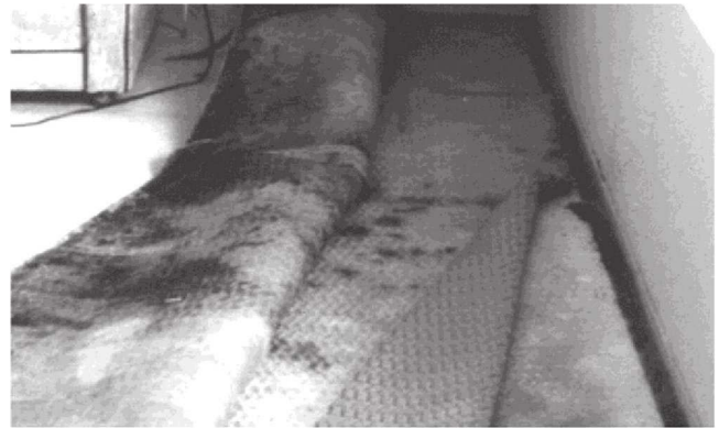
Fig. 1.3d—Mold growth in carpet due to moisture in concrete (photo courtesy of Floor Seal Technology, Inc.).
