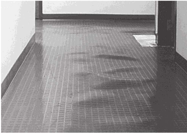
Fig. 1.3a—Debonded sheet flooring due to moisture in the concrete slab (photo courtesy of P. Craig and H. Protze III).
