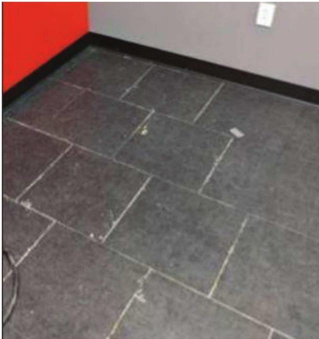
Fig. 1.3b—Adhesive bleed (image courtesy of Adam Bakeman).
