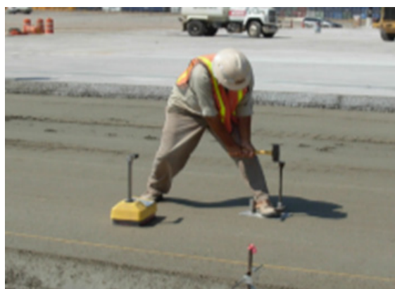
Fig. 4—Driving the pilot hole pin. (Figure courtesy of Portland Cement Association.)
