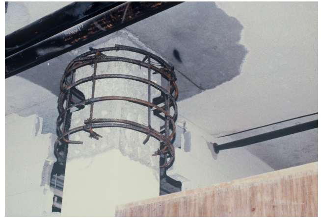
Fig. 3—Section enlargement of column with collar.
