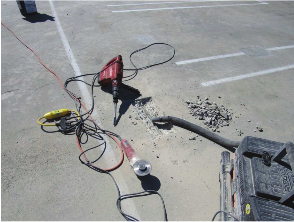
Fig. 1—Ongoing concrete removal operation in a post-tensioned slab using a lightweight electric impact breaker (photo courtesy of Wiss, Janney, Elstner Associates, Inc.).
