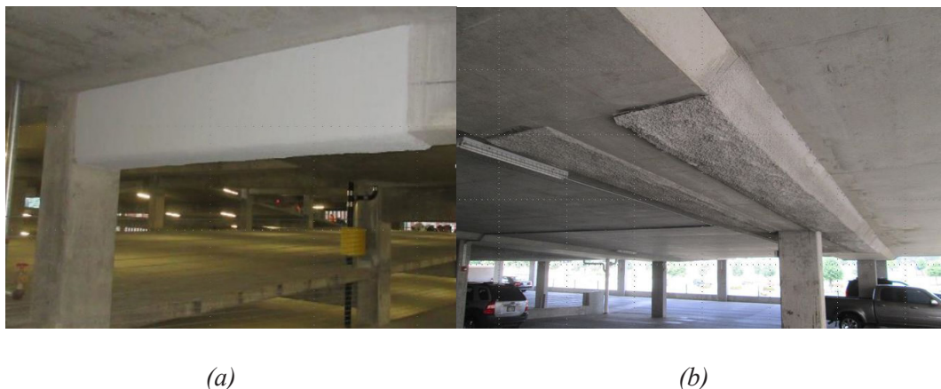
Fig. 1—Examples of fire protection systems: (a) protective coating on shear repair; and (b) protective mortar on flexural FRP-strengthened members (images courtesy of M. Lee).
