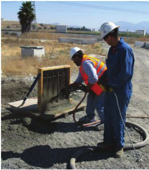
Fig. 1.6.3.3—Shooting certification panel with reinforcement.
