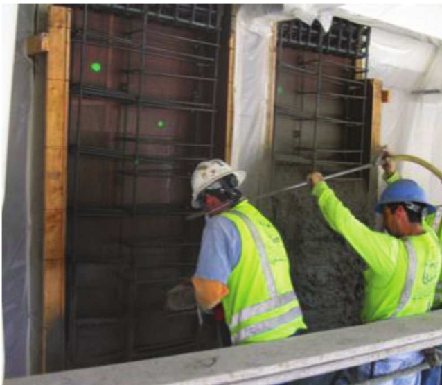
Fig. 1.5.1b—Crew shooting mockup panel.
