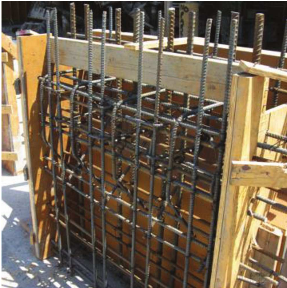
Fig. 1.5.1a—Typical example of mockup for evaluation of reinforcement encasement.
