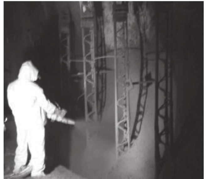
Fig. 5.5c—Typical lattice girder during shooting (manual).
