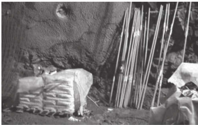
Fig. 5.2b—Rock bolts and grout.
