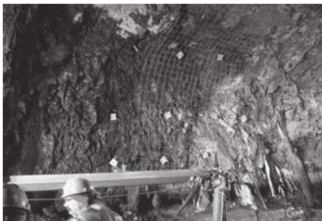
Fig. 5.3.2—Wire mesh in tunnel with considerable overbreak.
