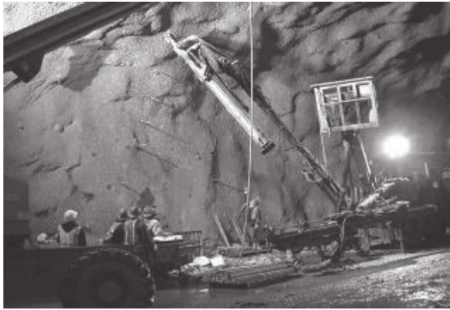
Fig. 5.2a—Rock bolt installation.
