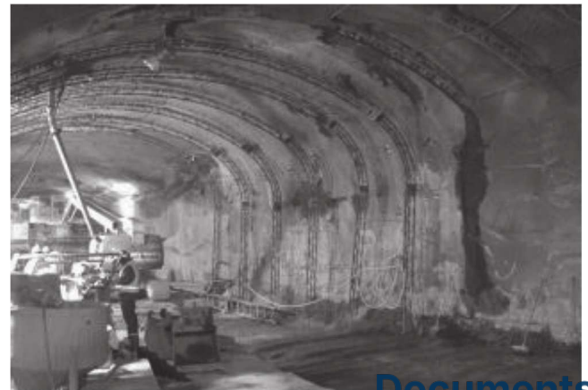
Fig. 5.5d—Tunnel with lattice girders.
