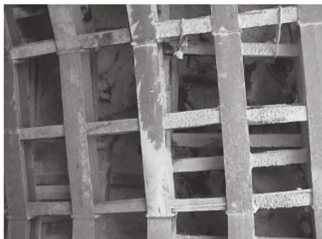
Fig. 5.6—Steel sets with significant wood cribbing.
