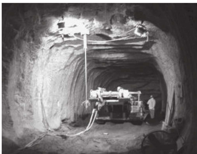
Fig. 1.1b—Typical heading: small tunnel with drill jumbo.
