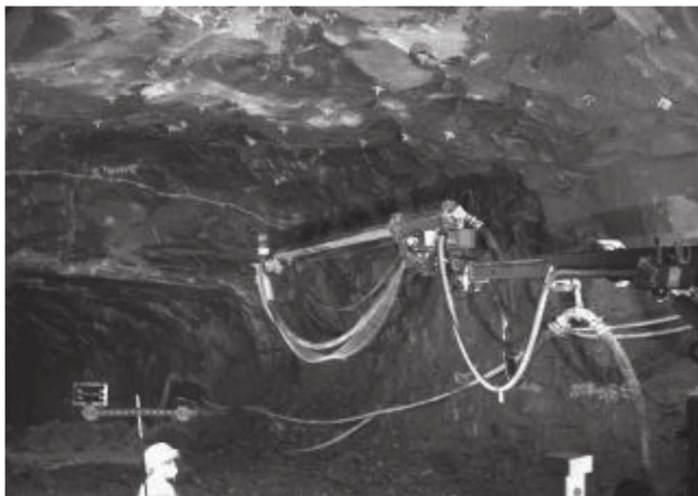
Fig. 5.2c—Tunnel with pattern bolting before shotcreting.
