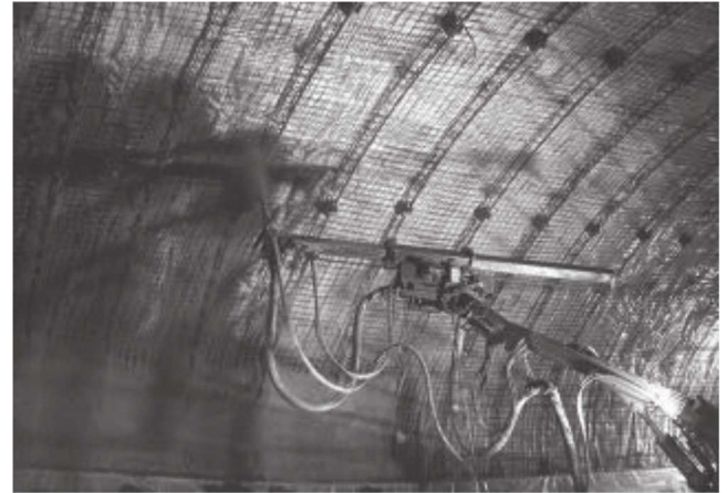
Fig. 5.5b—Typical lattice girder during shooting (robotic).
