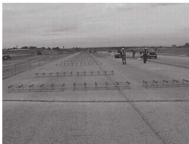
Fig. 3.3.2—Pervious concrete base prior to conventional paving at Lambert International Airport.
