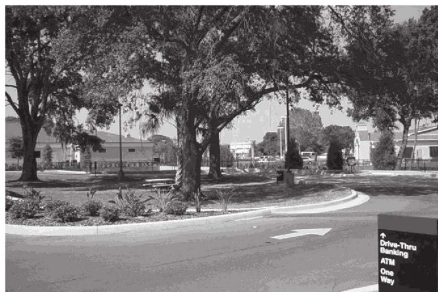
Fig. 3.3.1—Pervious concrete pavement used within the drip line of trees (photo courtesy of M. Offenberger).
