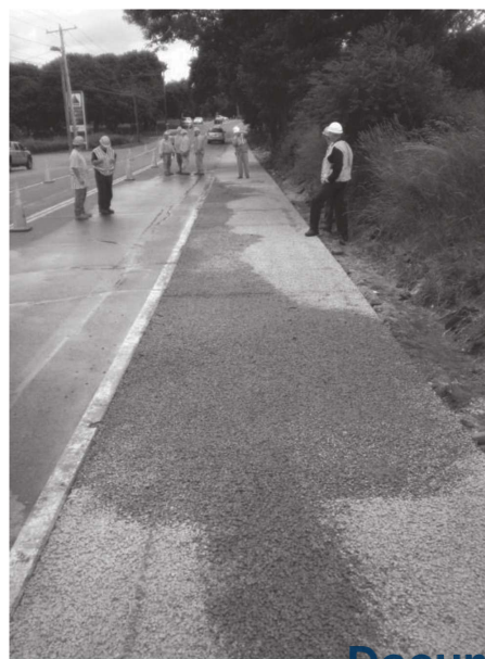
Fig. 3.3.3—Pervious concrete shoulder for flood control
