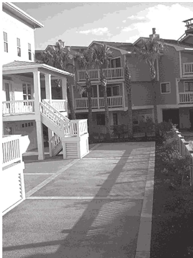
Fig. 3.1—Parking lot built with pervious concrete pavement.
