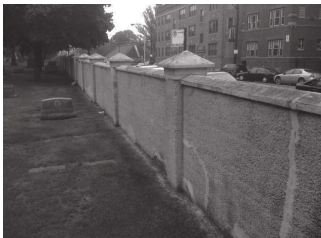
Fig. 3.2—Reinforced pervious concrete walls constructed in the early 1900s (photo courtesy of G. Seegebrecht).
