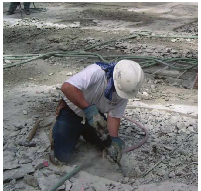
Fig. 4.2.3.1b—Handheld concrete breaker used to remove concrete around exposed reinforcement.
