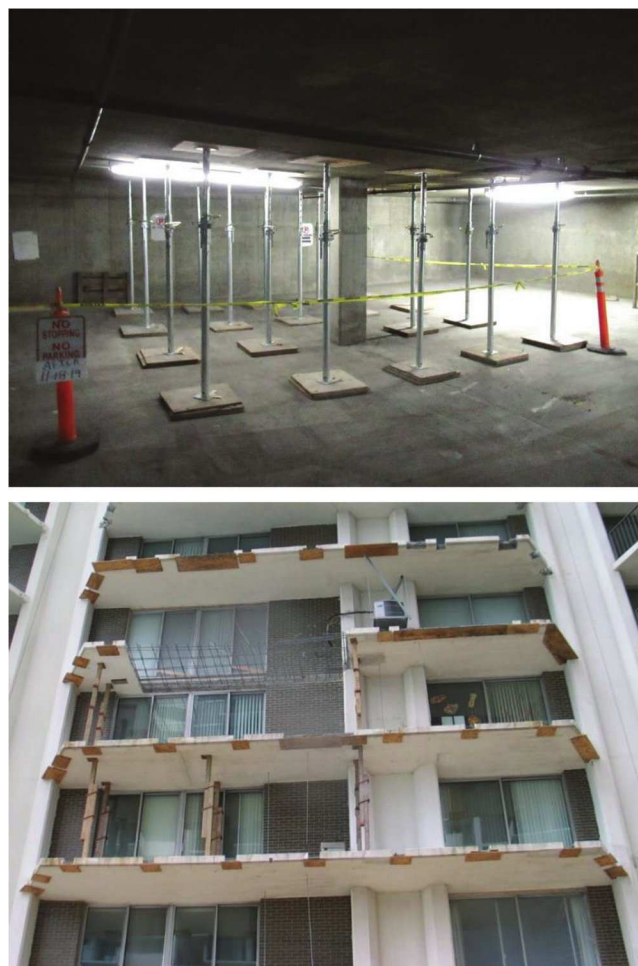
Fig. 4.2.2—Temporary shoring partitioning of garage floor (top) and balcony slabs (bottom).
