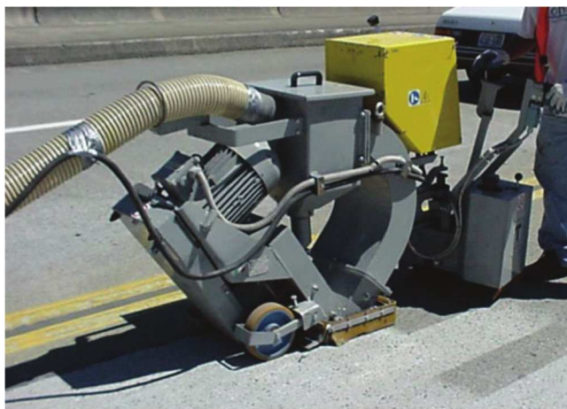
Fig. 4.3.2b—Shotblasting.
