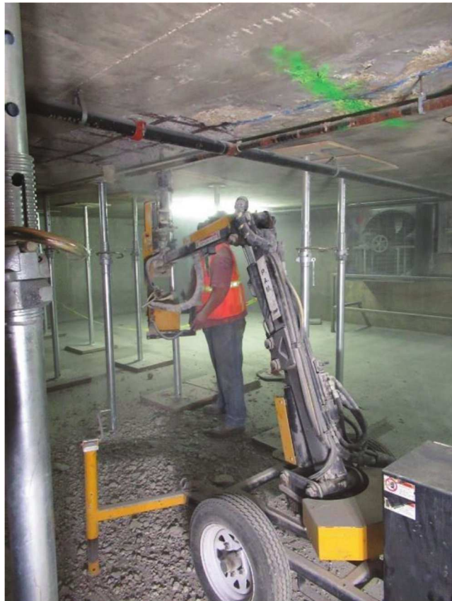
Fig. 4.2.4b—Boom-mounted concrete breaker used for underside repair.
