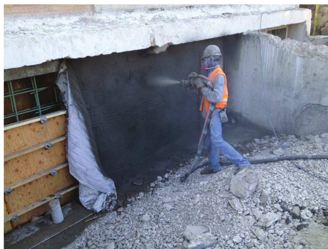
Fig. 3.2.2.3—Shotcrete placement. (Courtesy of Wiss, Janney, Elstner Associates, Inc.)
