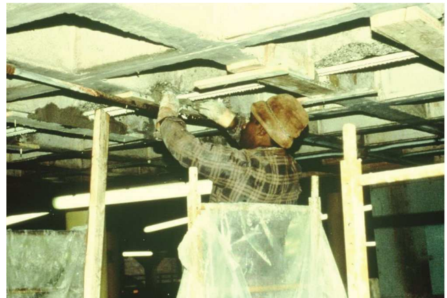
Fig. 3.2.2.1b—Form-and-drypack overhead placement (courtesy of Wiss, Janney, Elstner Associates, Inc.).
