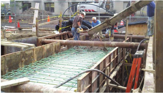
Fig. 3.6.1—Concrete being placed. (Courtesy of Wiss, Janney, Elstner Associates, Inc.)
