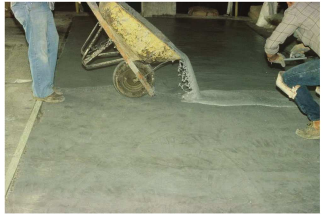
Fig. 3.3—Shallow overlay placement. (Courtesy of Wiss, Janney, Elstner Associates, Inc.)
