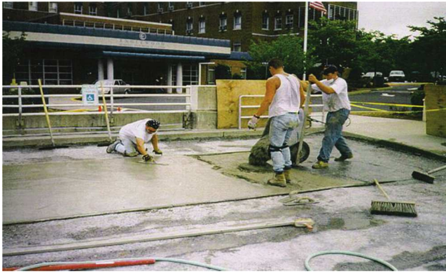
Fig. 3.2.1—Placement of concrete overlay. (Courtesy of Euclid Chemical Company.)
