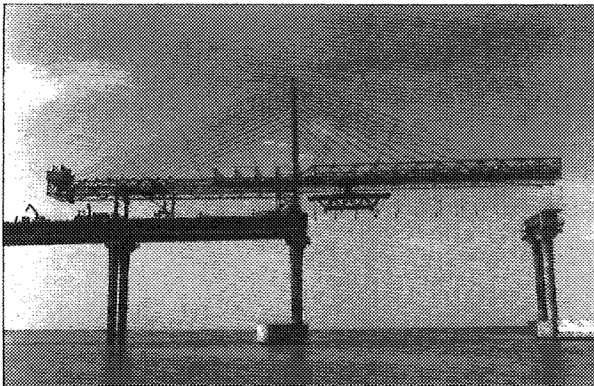
Figure 12: Bubiyan bridge, The erection beam, placing the first segment of the main span (photo M. V.).
