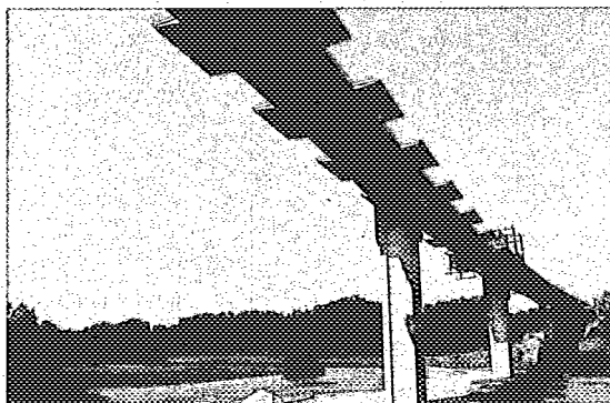
Figure 25: The Arrêt Darré viaduct. Construction in situ of the lateral parts of the top slab (photo Cl. Servant).
