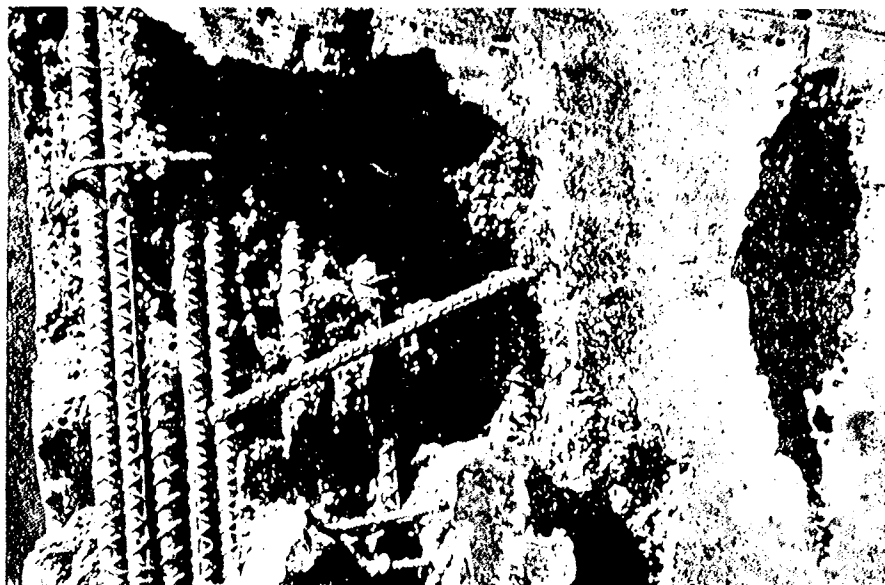
Fig. 1-6 Congested reinforcement is the principal cause of the sand pockets and porous areas shown here. Such design and placement of reinforcement is not recommended even for conventional concreting; in shotcrete construction it is impossible to get sound material between and behind the bars.
