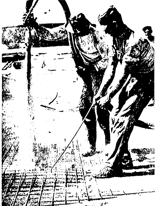
Fig. 2-8 Shooting a tank floor. Reinforcement is pulled up so that it will be as close as possible to the center of the slab.
