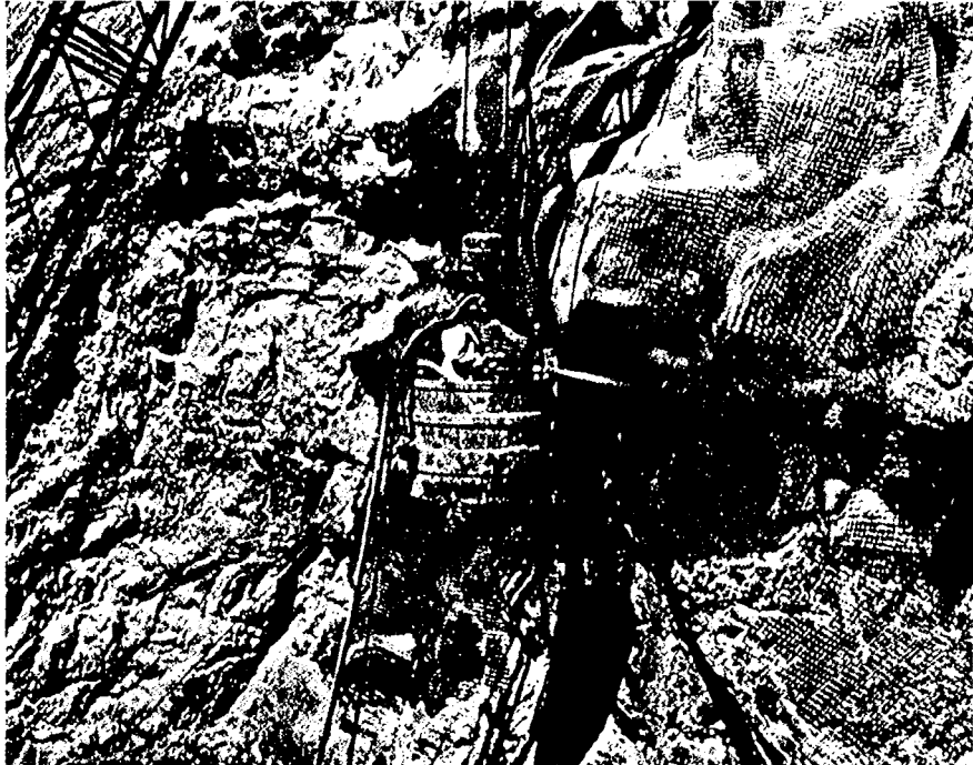
Fig. 1-2 Shotcrete can readily be placed in many locations virtually inaccessible for conventional concreting. One example is this rock stabilization work.
