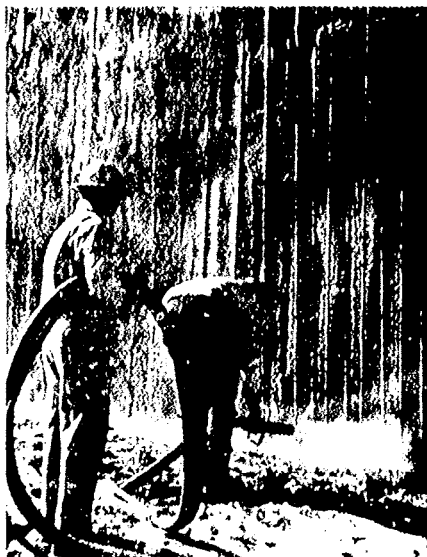
Fig. 2-5 Nozzle held low to shoot base of wall, but not so low as to pick up sand from ground. Hose-dragger leaves 3 or 4 ft of slack hose on ground immediately behind nozzleman for ease of handling by nozzleman.
