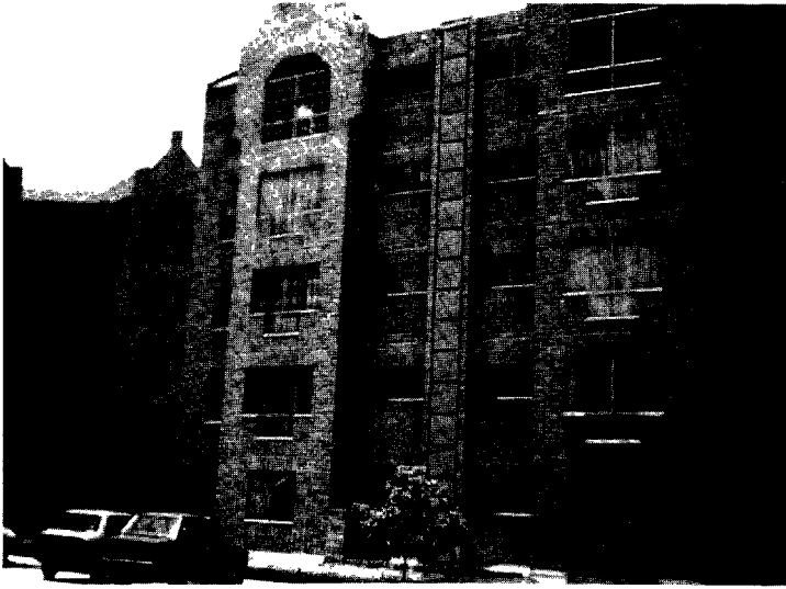
Fig. 5b—Masonry building in Latin America — Peru
