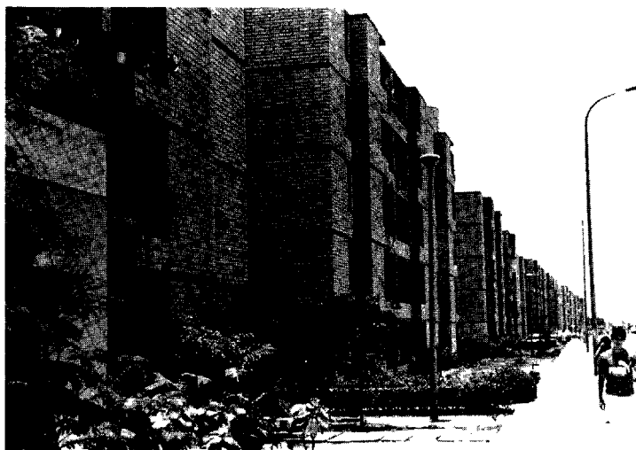
Fig. 5a—Masonry building in Latin America — Colombia
