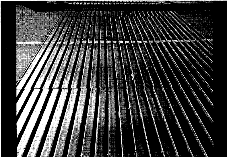
Fig. 18—Modular system for very large movements—Tagus Bridge in Portugal
