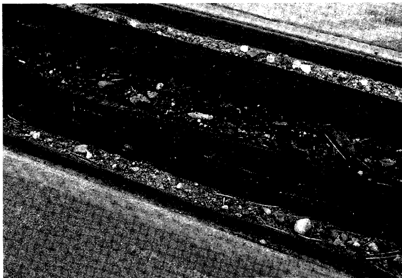
Fig. 10—Typical attrition to elastomeric wearing surface—Delastaflex
