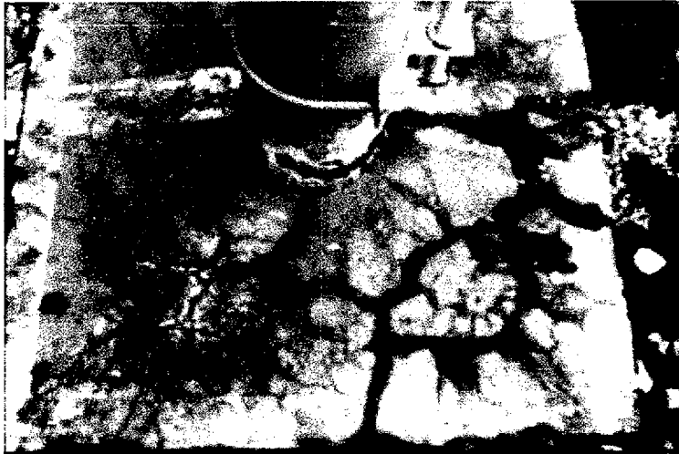
Fig. 4—Cracking in cast-in-situ concrete pedestal for electric power line.
