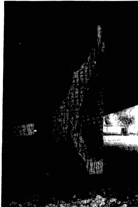
Fig. 5—Shear distress pattern at I-10, Fairfax and Washington.
