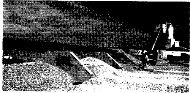
Fig. 4.1—Aggregate piles must be kept clean and separate. Minimize segregation.
