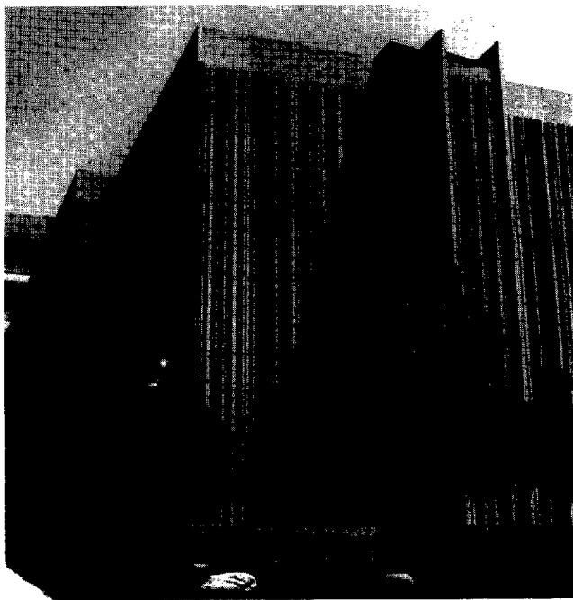
Fig. 1.4—Building design accented with vertical patterns and joints; quality construction provides a highly functional and aesthetic workplace.
