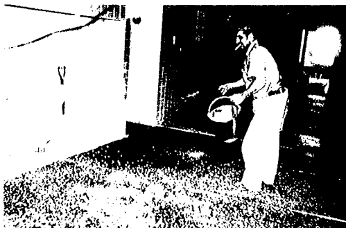
FIG. 4-3 SPRINKLING AGGREGATE ON TERRAZZO TOPPING
