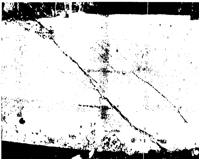
FIG. 5-1 CRACKED CONCRETE SEAT BEAM PRIOR TO REPAIR
