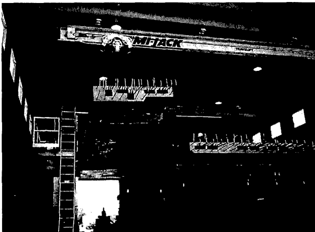
Figure 11. Positioning of segments by crane prior to bonding together
