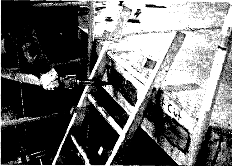
Figure 13. Grouting of post-tensioning ducts
