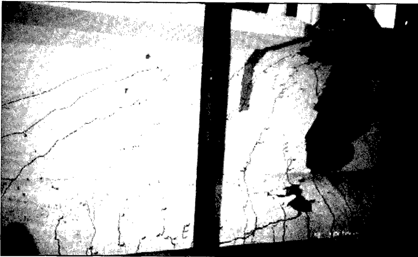
Figure 6 A View of Type V Girder after Failure
