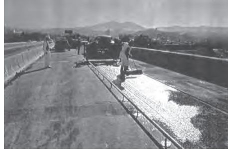
Figure 6: Application of the primer.
