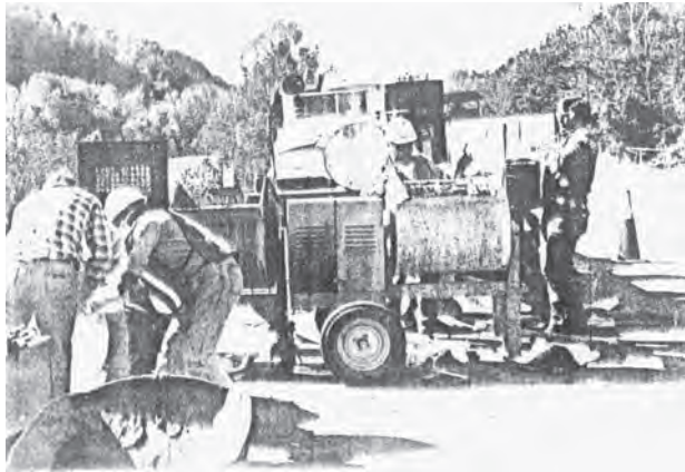
Figure 6. Mixing the electrically conductive PC overlay composite.
