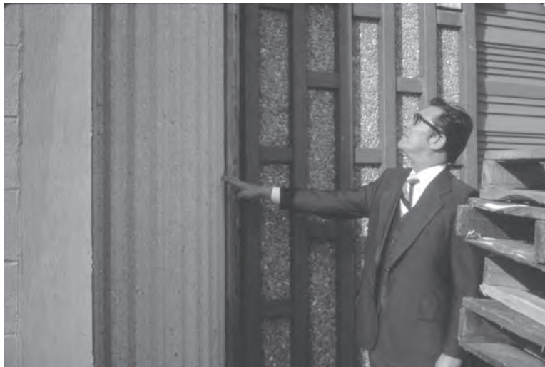
Figure 1: Precast Wall Panels (courtesy of Prusinski).
