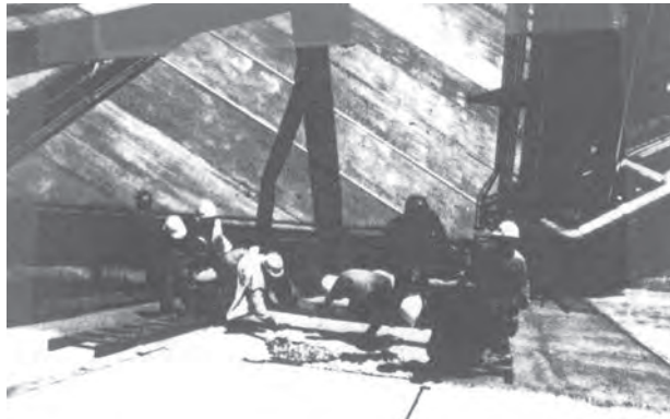
Figure 1. Installing IPC overlay on sloped walls of containment dike.
