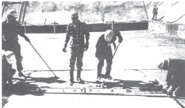
Figure 2. Vibrating screed used to finish IPC overlay.
