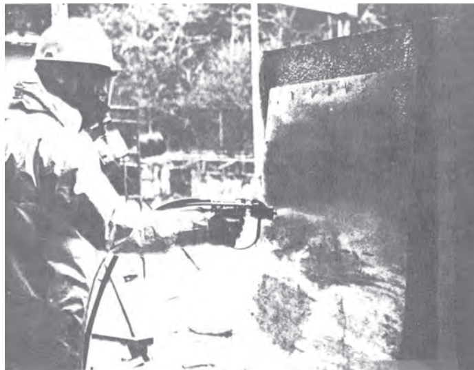
Figure 5. Spray application of electrically conductive coating.
