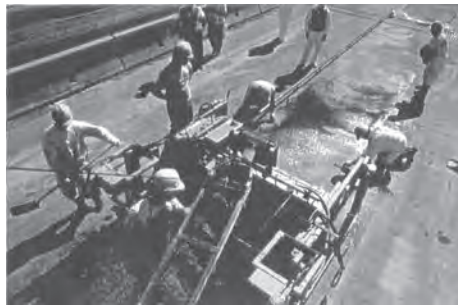
Figure 7: Automated deposition of the premixed polymer concrete.
