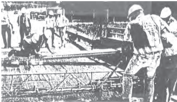
Figure 7. Screeding the electrically conductive PC overlay.
