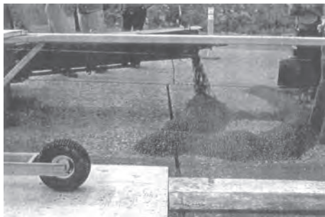
Figure 3: Spreading of the premixed polymer concrete.
