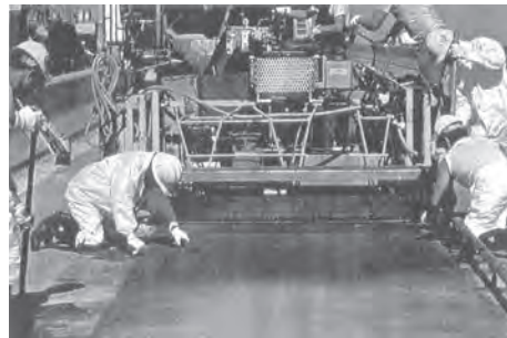
Figure 8: Inspection of placed 3/4 inch overlay.
