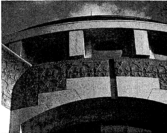
Fig 7 1670 sq.m of GFRP panels on the Cervantes Convention Centre, St Louis, Missouri. 2 finishes – Ornate/pigmented and stone simulation
