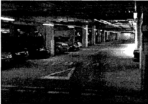
Figure 8. General view of a typical basement car park. Note transverse cracks in floor in foreground.
