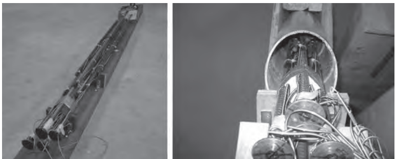
Figure 8 – Preparation of the stud reinforcement and placement inside the FRP tube
