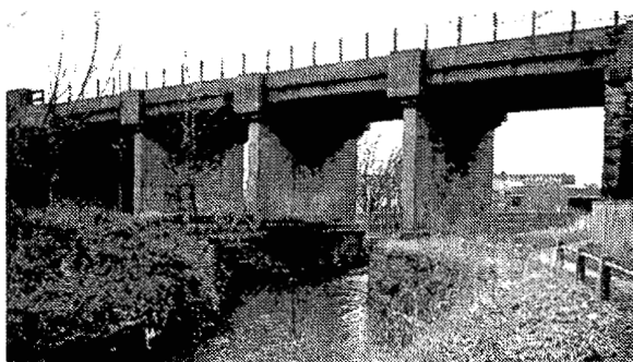
Figure 14 - Adam Viaduct, Wigan
