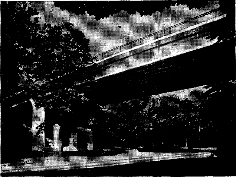
Figure 11 – Walnut Lane Bridge in Philadelphia
