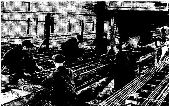
Figure 7 - Original long-line prestressing beds for railway sleepers 13 .
