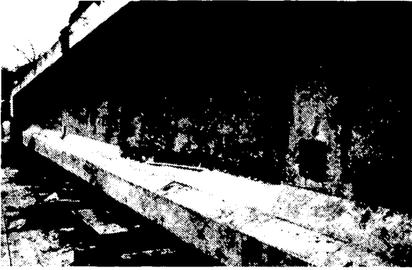
Figure 13 – Honeycombs in the first girder cast in 1949
