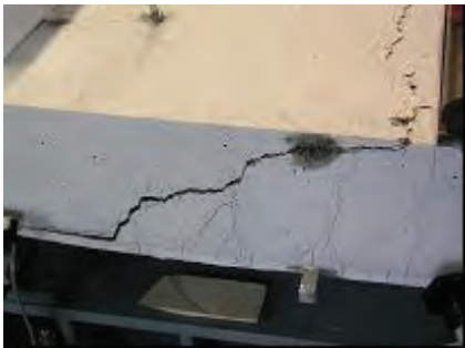
Figure 12 — Failure of the component due to flexural shear stresses
