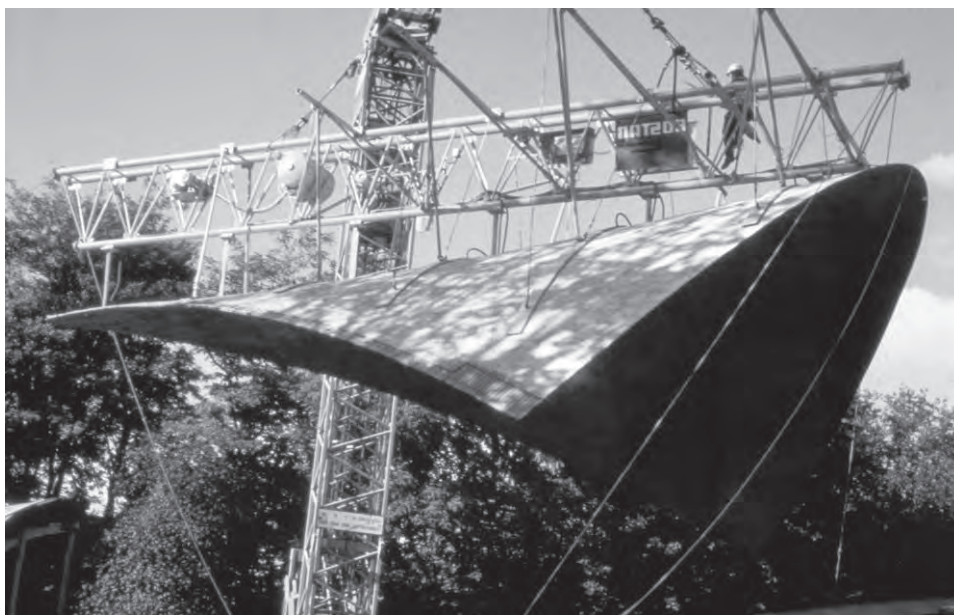
Fig. 14 — One of the eight GRC elements by Schlaich during the assembly
