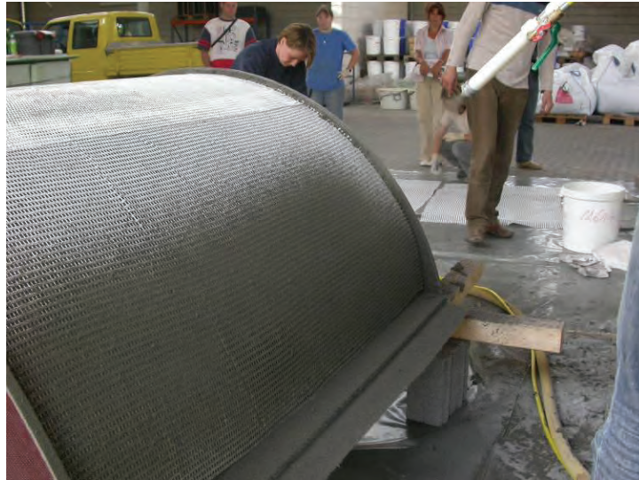
Fig. 2 — Shotcrete applied on the semi-cylindrical barrel shell
