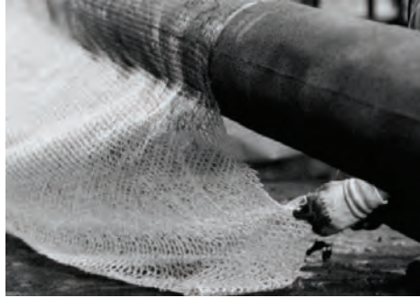
(a) Retrofitting of steel-reinforced concrete piles by textile-reinforced concrete
