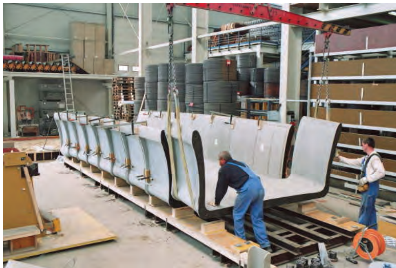
Fig. 8 — Segmented, prestressed pedestrian bridge at the University of Dresden
