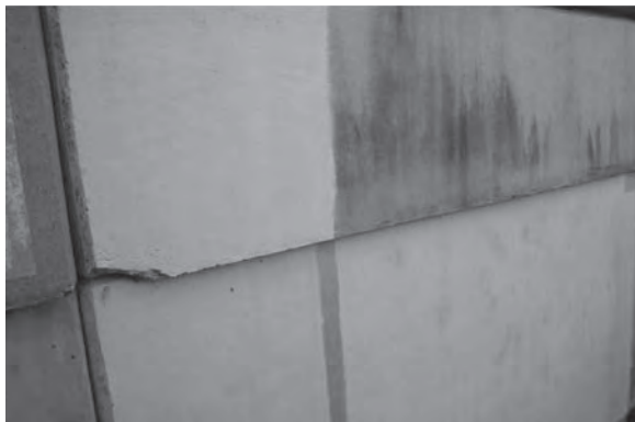
Fig. 4—Self-cleaning coating made of nano-particles. [13]
