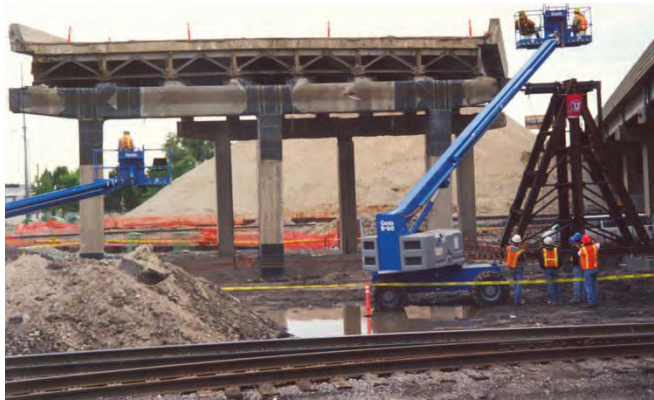
Figure 7 - In-situ lateral load test of bridge pier – 1998 tests.
