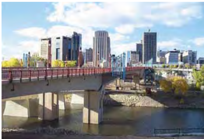
Fig. 3—Wabasha Street Bridge, Minneapolis-St. Paul, MN; 75% slag-cement concrete in pier foundations, 65% in pier stems; 1996-1998.
