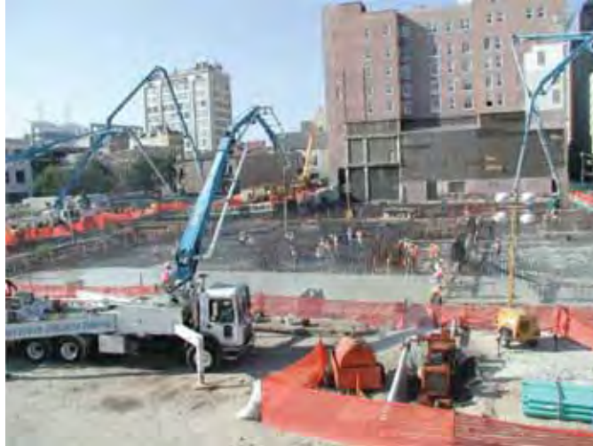
Fig. 8—RSA Battle House Tower, Mobile, AL; 60% slag-cement concrete; 23-h placement starting November 7, 2003.
