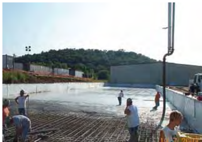
Fig. 7—JTM freezer floor placement, Harrison, OH; 60% slag-cement concrete; night placement ending in morning, July 2003.
