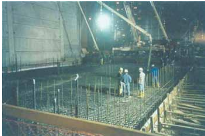
Fig. 6—Express Parking Structure, Indianapolis, IN; during night placement beginning on February 26, 2000; 70% slag-cement concrete
