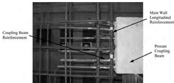
Fig. 1—Precast coupling beam embedment detail.
