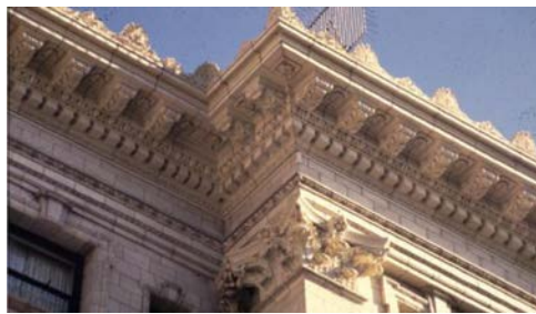
Fig. 12—GFRC replacement cornice, Fairmont Hotel, San Francisco.
