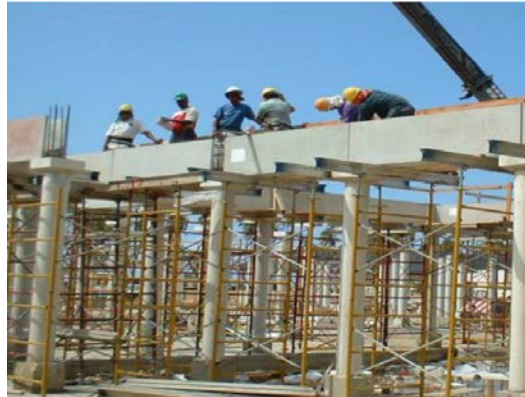
Fig. 28—GFRC beam forms placed between column forms before pouring concrete.
