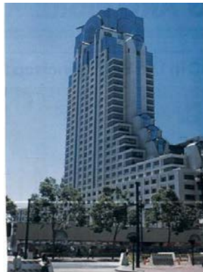
Fig. 10—Biege GFRC panels cladding Marriott Hotel, San Francisco.
