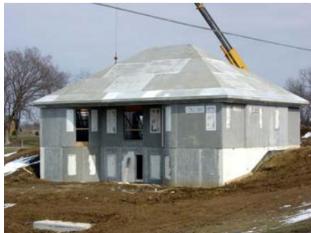
Fig. 16—GFRC house under construction.
