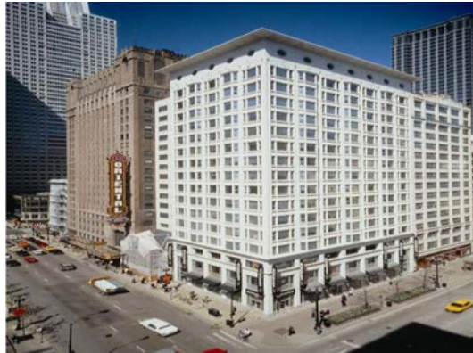
Fig. 9—White GFRC panels cladding Art Institute, Chicago.
