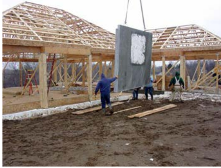
Fig. 14—Installation of insulated GFRC wall panel.
