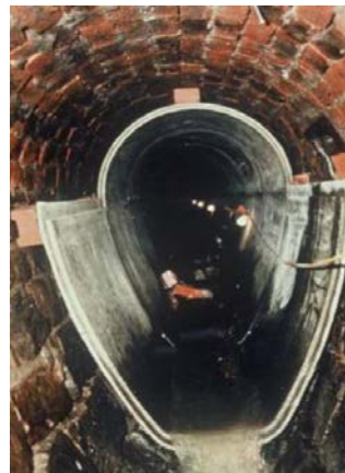
Fig. 18—GFRC panels relining old brick sewer, London, UK.
