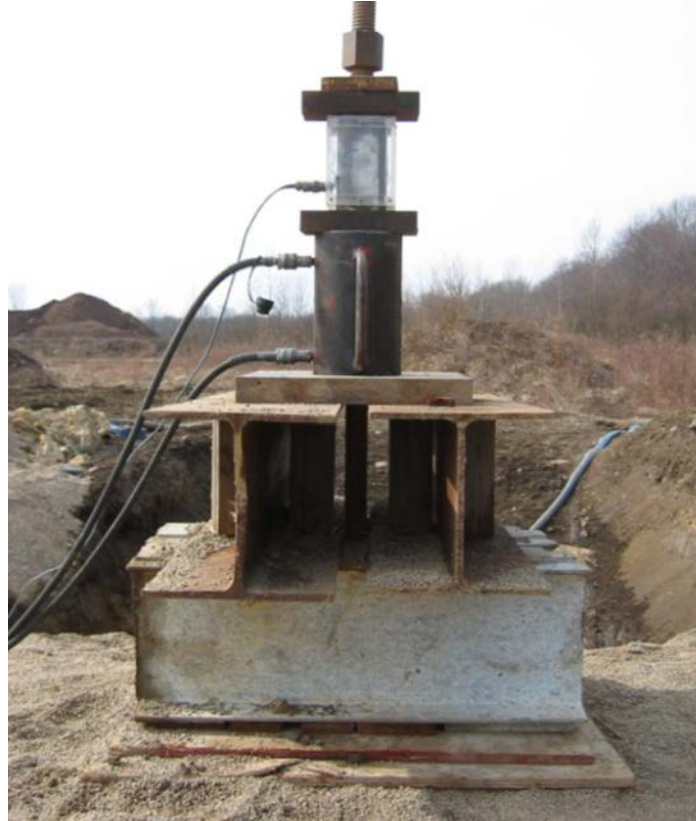
Fig. 9—Load jack and loading block set above top of arch with 1 ft. (305 mm) earth cover.
