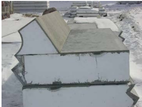
Fig. 15—Insulated GFRC roof panels showing joint design.
