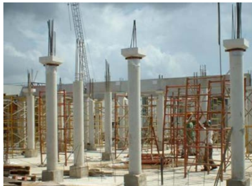
Fig. 27—GFRC column forms in place.
