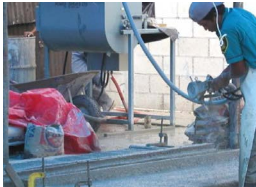
Fig. 23—Spraying GFRC onto steel mold. After spraying mold, sides are folded vertically and secured.
