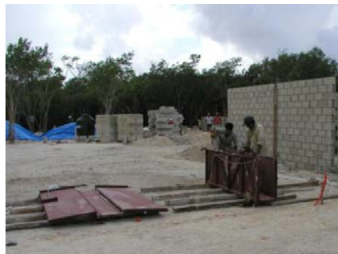
Fig. 21—Steel folding forms for GFRF beam forms.
