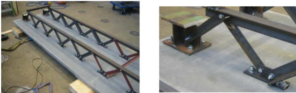
Fig. 8—Steel truss assembly and bolted connection to ECC slab.
