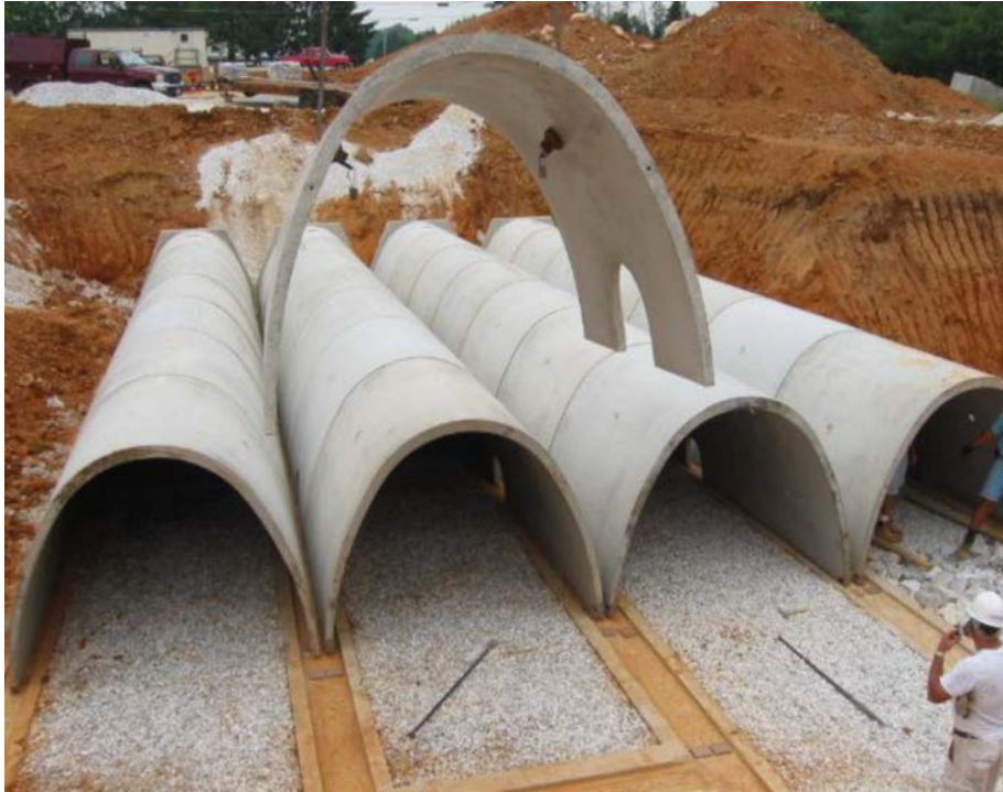
Fig. 13—Application of SFRC arch unit for stormwater detention facility.
