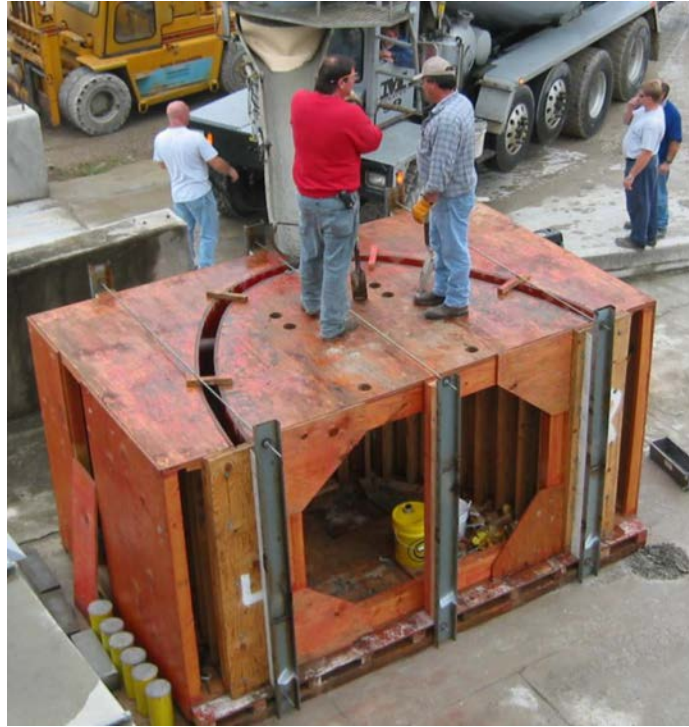
Fig. 7—Wood form for precast SFRC arch unit.
