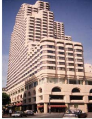
Fig. 11—Biege GFRC panels cladding Park Plaza Hotel, San Francisco.
