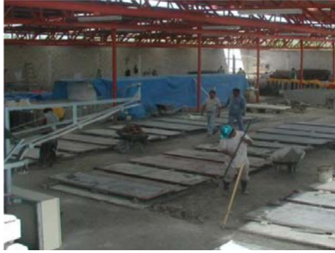
Fig. 22—Lay-out of steel folding forms in the factory.
