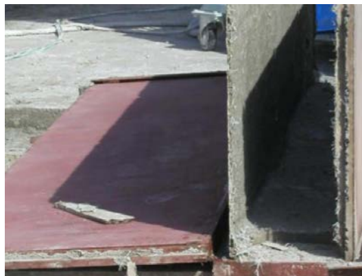
Fig. 24—Demolding by dropping sides of steel mold. GFRC unit then removed.
