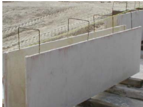
Fig. 20—GFRF permanent beam form.
