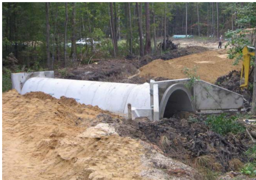
Fig. 14—Application of SFRC arch unit for stream crossing.
