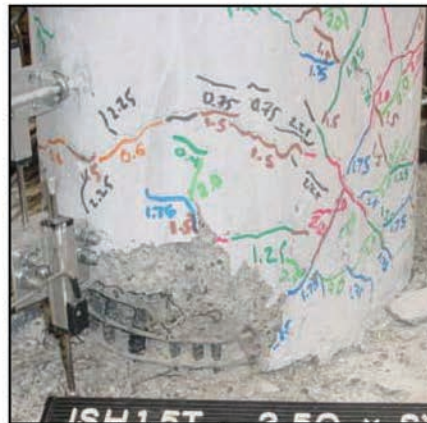
DS-5: imminent failure
