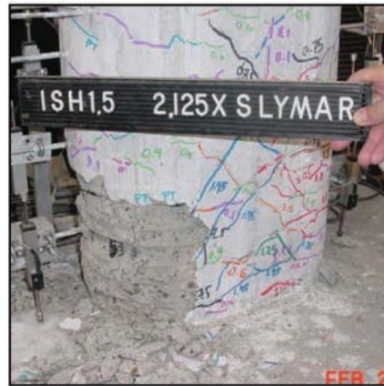
DS-4: lateral and longitudinal bars visible
