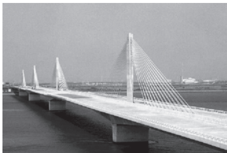
Fig. 23—Kiso River Bridge.
