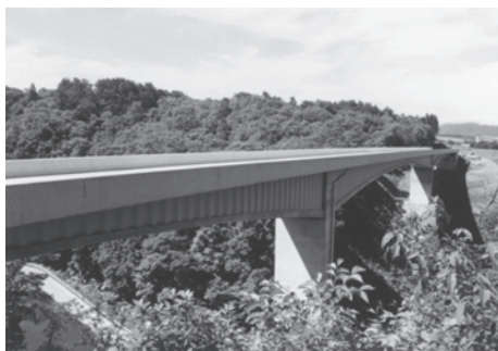
Fig. 16—Hontani Bridge with corrugated web.
