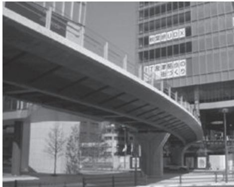
Fig. 21—Pedestrian bridge in Akihabara constructed with UHSC.
