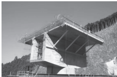
Fig. 26—PS box girder with inclined struts.
