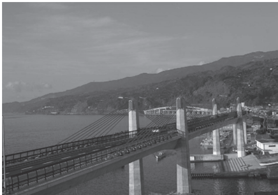
Fig. 14—Odawara Blue Way Bridge (three-span continuous extradosed PS bridge).
