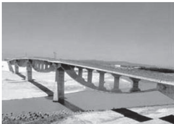
Fig. 27—Shiosai Bridge (four-span continuous stress-ribbon PS bridge).
