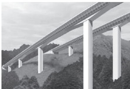
Fig. 25—Shibakawa Viaduct (continuous PS box girder with inclined struts).
