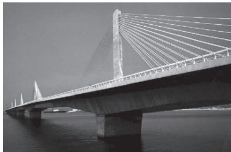
Fig. 24—Ibi River Bridge.
